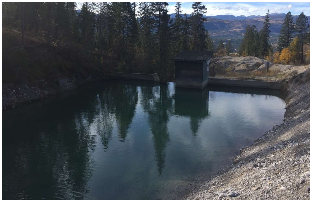
Photo 2: The reservoir with the debris removed. October 21, 2021.
