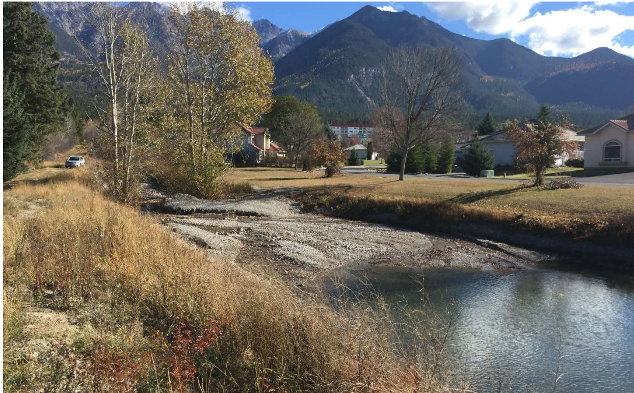
Photo 5: The lower debris trap near completion of debris removal. December 4, 2020.
