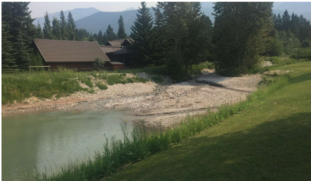
Photo 4: The lower debris trap after the May 24 event. July 15, 2021. The material deposition was minor and the material was not removed.
