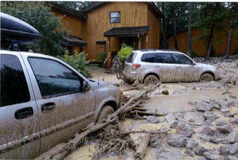
Damage to Mountainside Villas, upper fan (Source A.B.)
