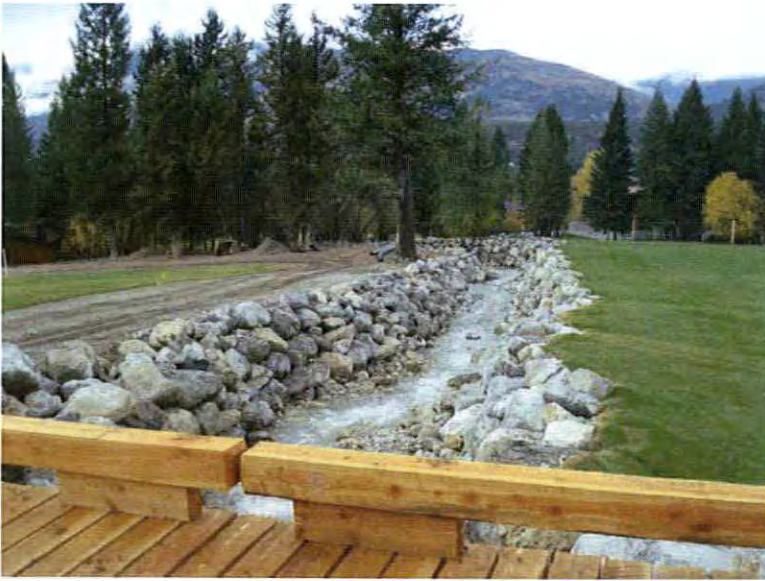
Channel, view downstream across 16 th Fairway
