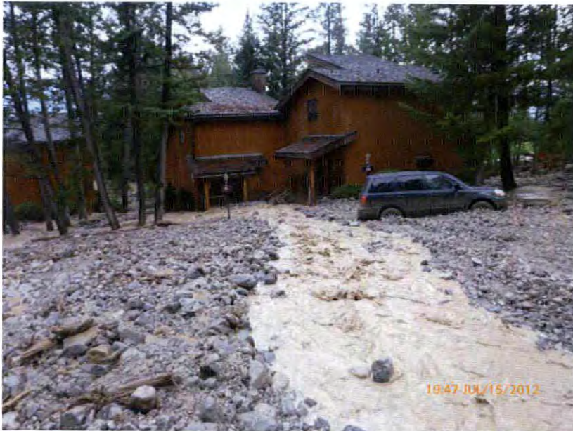
Deposition at Mountainside Villas, upper fan (Source A.B.)
