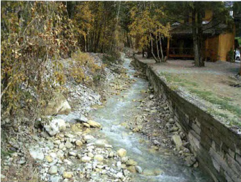
Channel near townhomes, contained on one side with wood crib wall (relatively undamaged in July) (Oct. 16, 2012)
