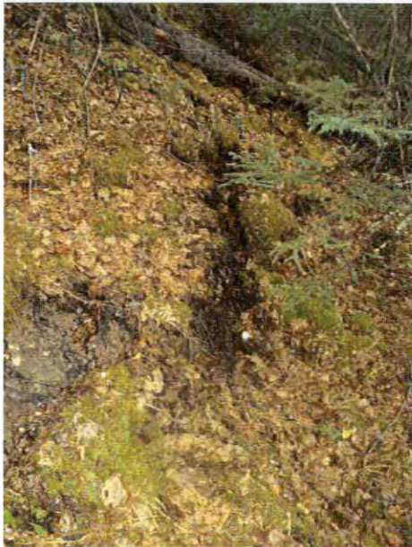
Tension cracks indicating slope instability above north tributary (Oct. 15, 2012)
