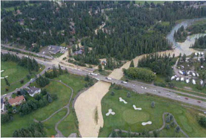
Aerial view showing flooding of Highway 93/95 (Source A.B.)
