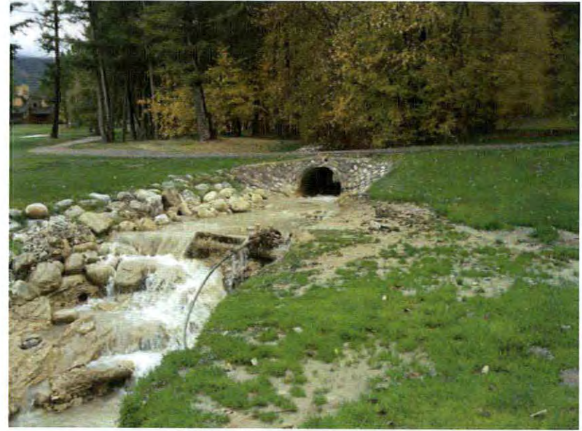
Culvert on Mountainside Golf Course, mid-fan below pond (Oct. 17)
