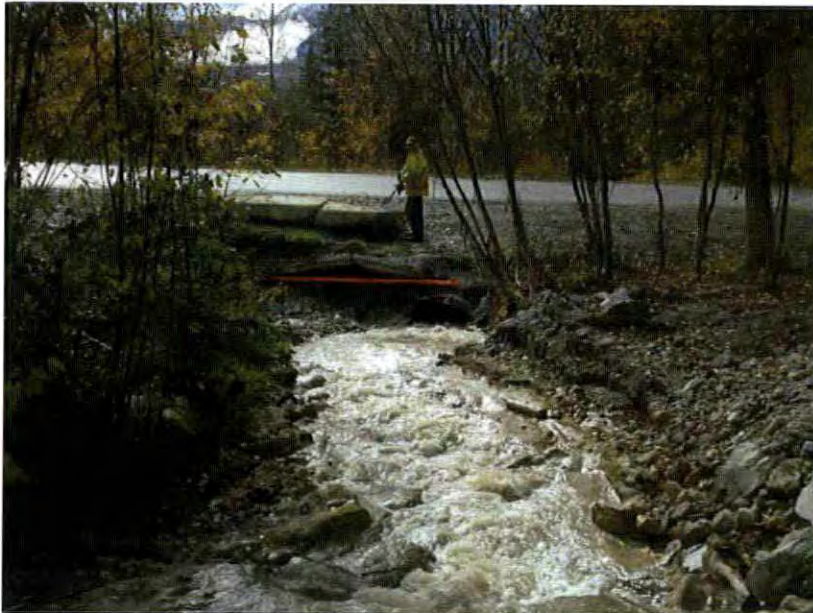
Culvert under road, upstream of mouth (Oct. 17, 2012)
