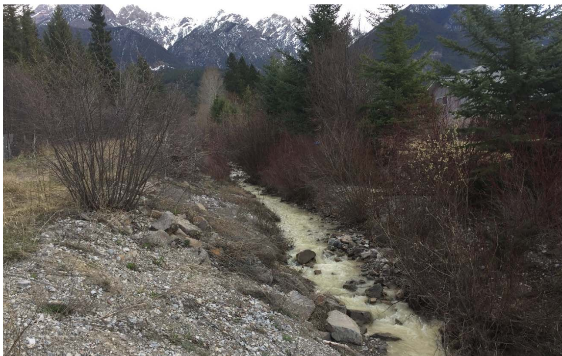
Photo 10: Channel immediately upstream of the lowest culvert. April 23, 2020.
