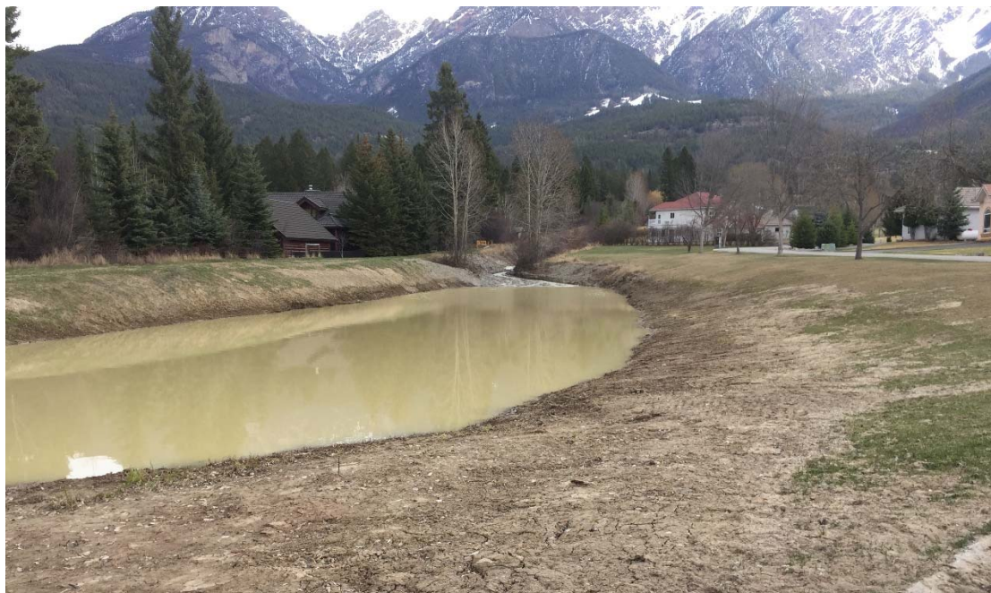
Photo 7: The lower debris trap, April 23, 2020.
