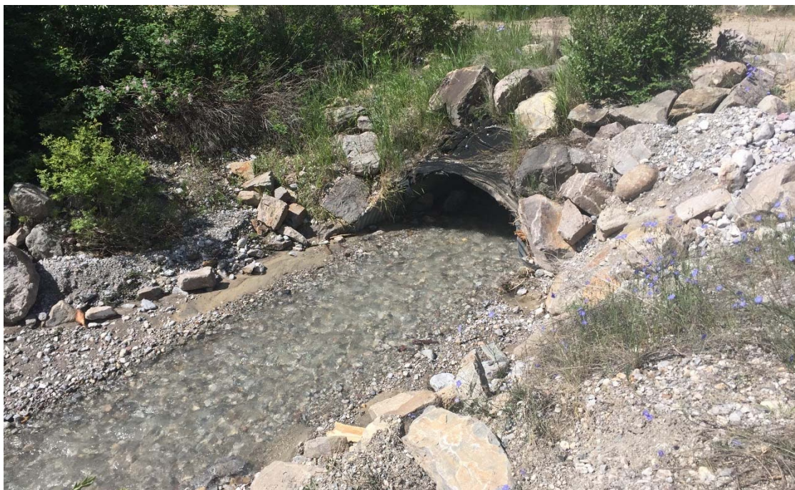
Photo 5: The culvert immediately upstream of the lower debris trap. June 10, 2020.
