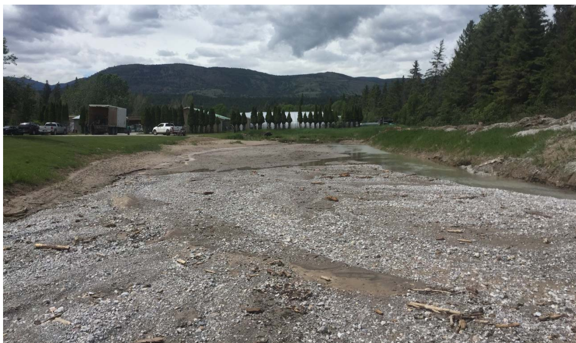
Photo 8: The lower debris trap after the May 31 event. June 9, 2020.
