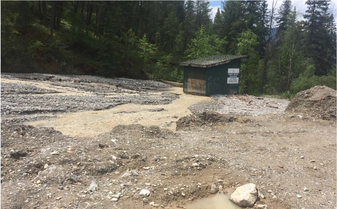
Photo 2: Cold Spring Creek Reservoir after the May 31 event. June 1, 2020.
