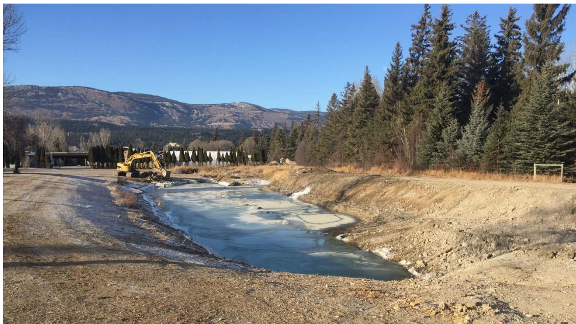
Photo 9: The lower debris trap near completion of debris removal. December 4, 2020.
