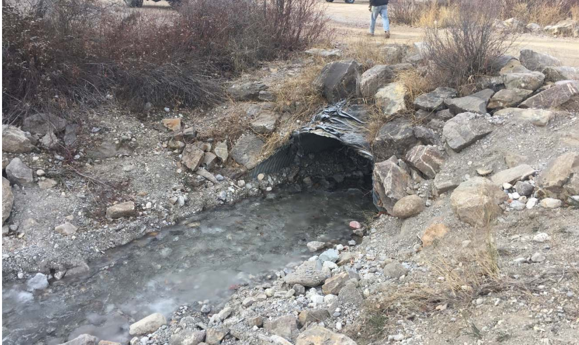
Photo 6: Culvert upstream of the debris trap after cleaning. November 30, 2020.
