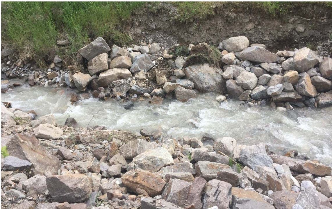
Photo 12: Repair of bank erosion. June 9, 2020.
