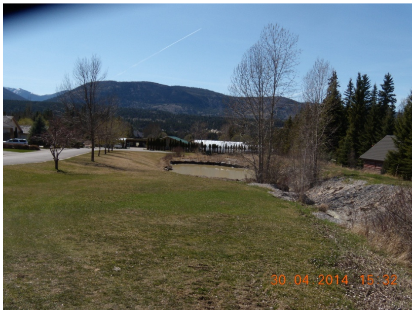
2014 conditions at the lower debris trap on Cold Spring Creek
