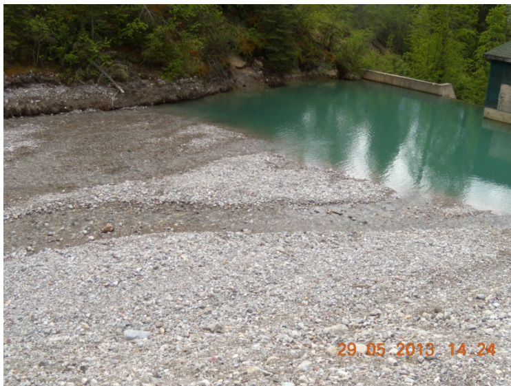
May 29, 2013 Reservoir Sediment Deposition
