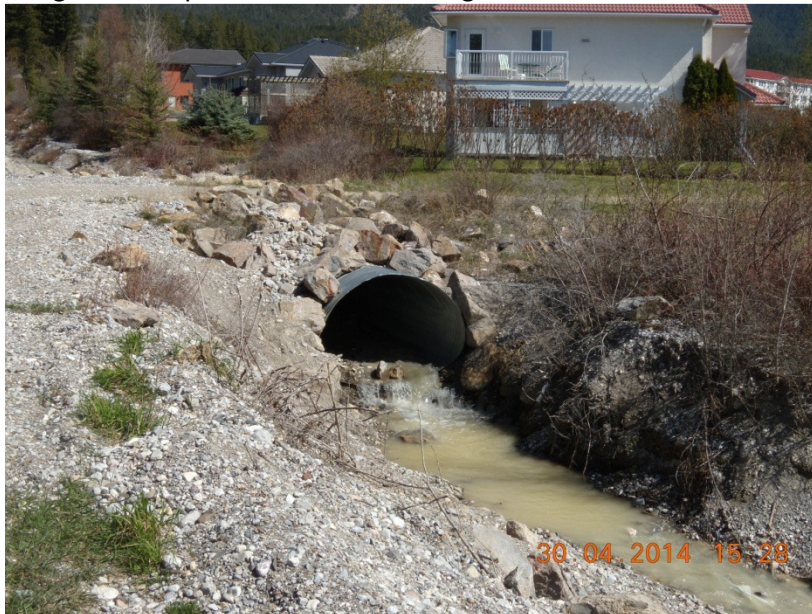
Culvert condition at the time of formal inspection April 30, 2014
