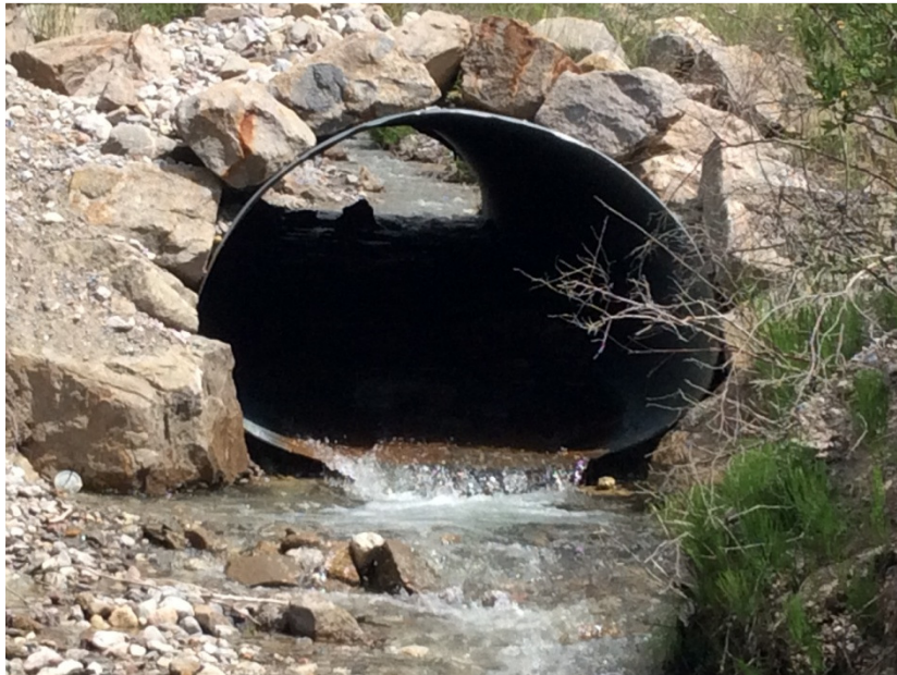
Culvert condition at the time of monitoring inspection June 24, 2014
