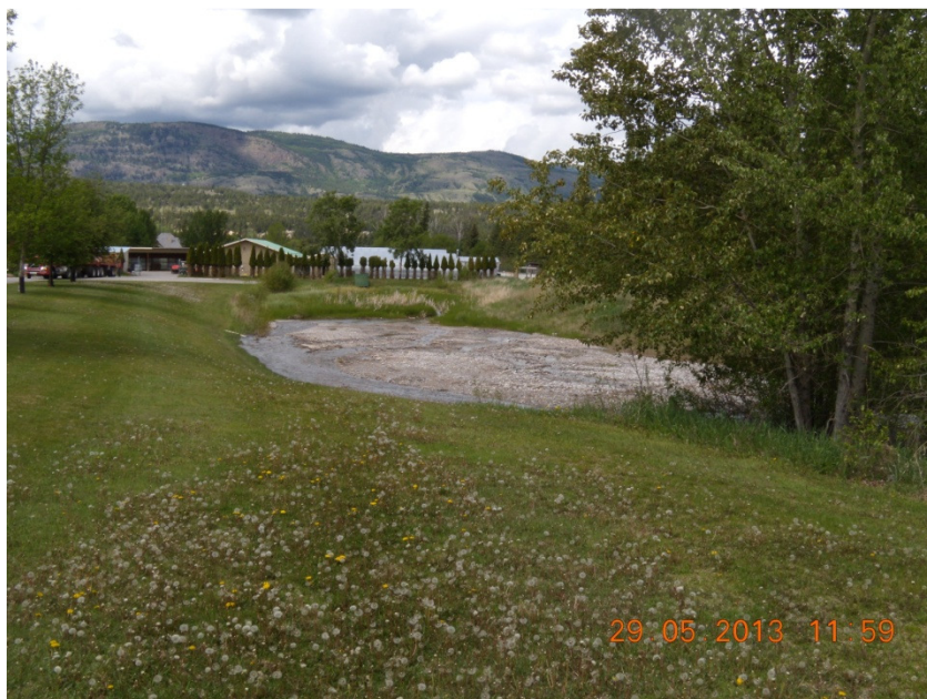
Debris Trap Sediment Deposition prior to the 2013 debris flow
