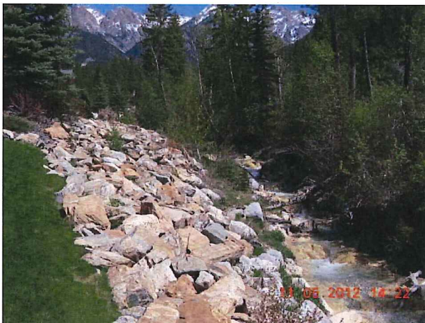
Pre-Debris Flow Event May 11, 2012 Site Conditions
