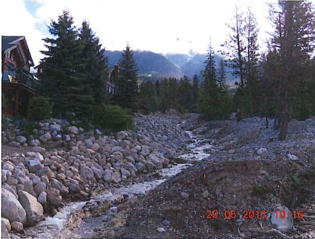
May 29, 2013 Dike/Site Conditions
