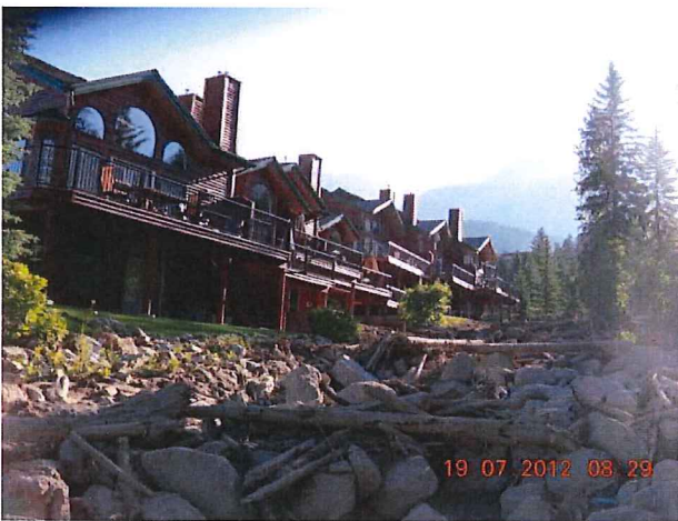
Post Debris Flow Event July 19, 2012 Dike Site Conditions
