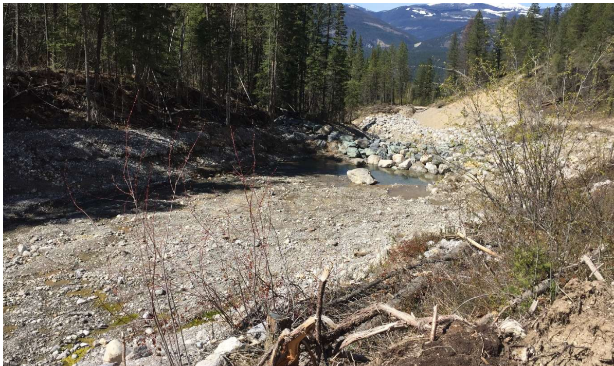
Photo 4: Weir 2 in good condition looking downstream. May 5, 2021.
