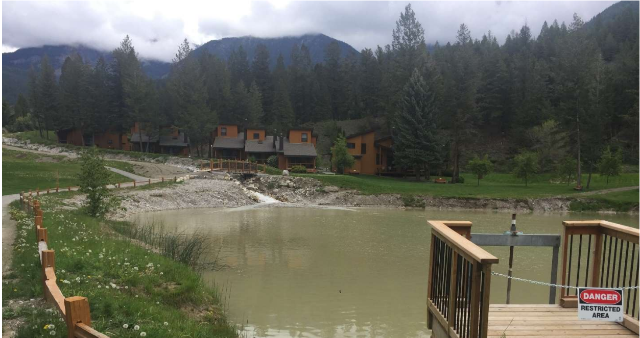
Photo 19: Hole 12 pond inlet with minimal deposition at the inlet. May 26, 2021.
