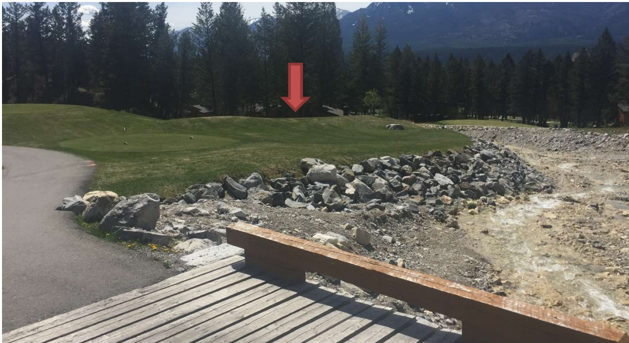
Photo 12: The left hand dike is in good condition. May 5, 2021.
