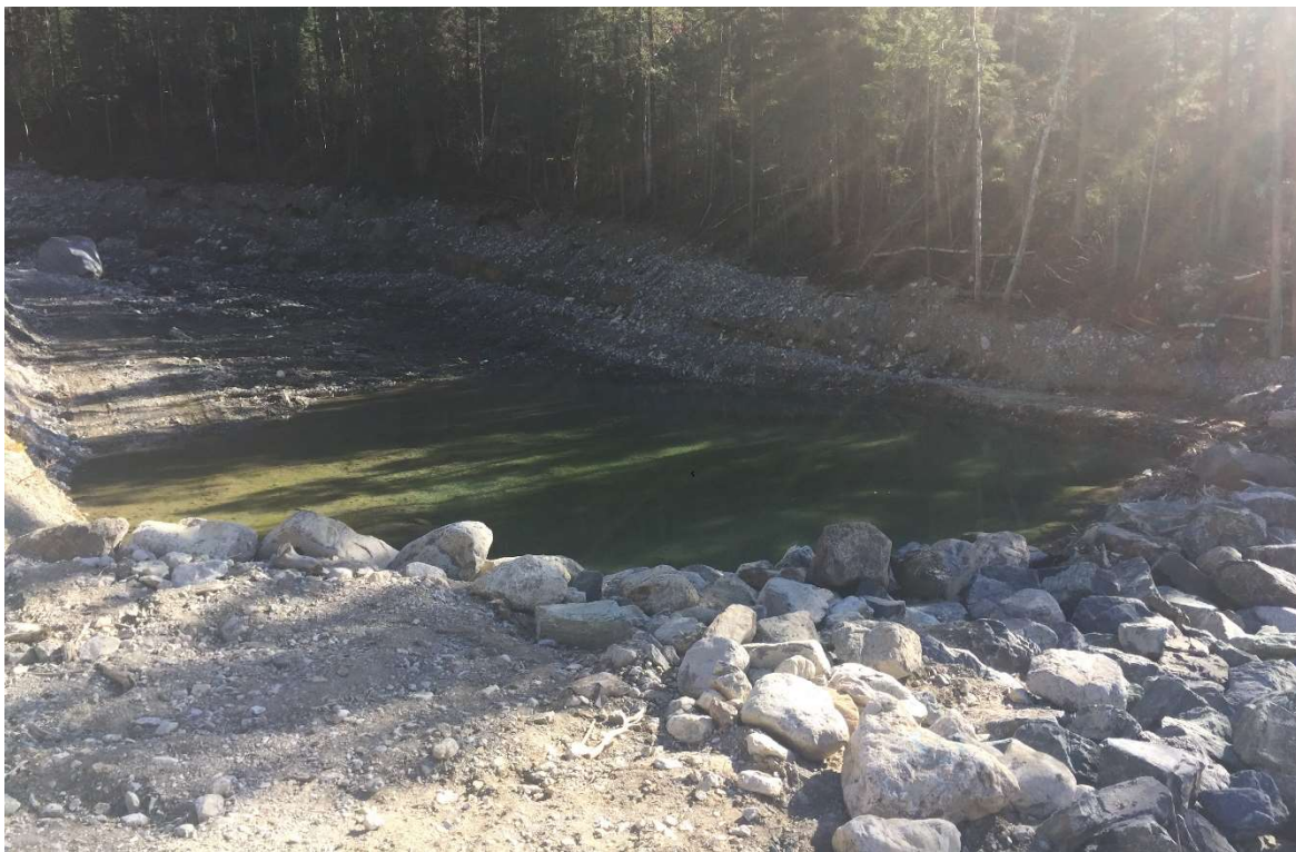
Photo 6: Weir 2 basin with debris flood material removed. October 21, 2021.
