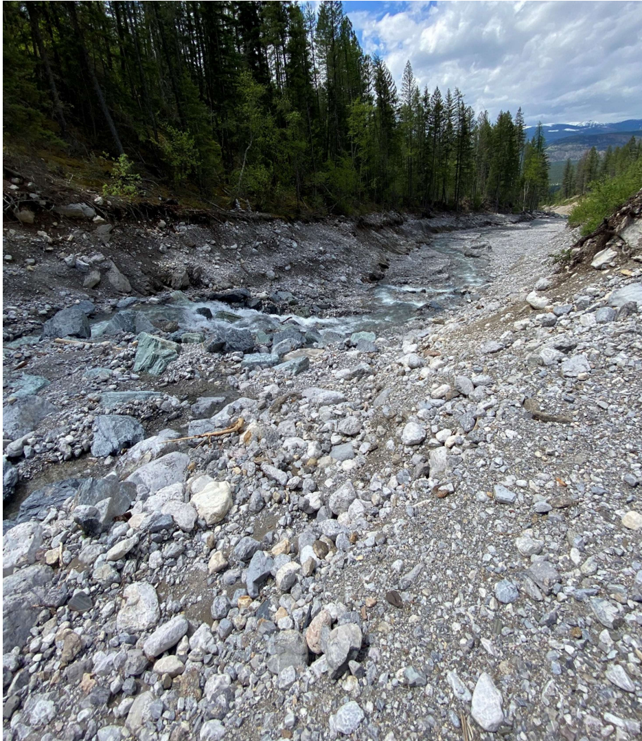
Photo 2: Weir 1, filled with debris material from the May 24 event. May 27, 2021.
