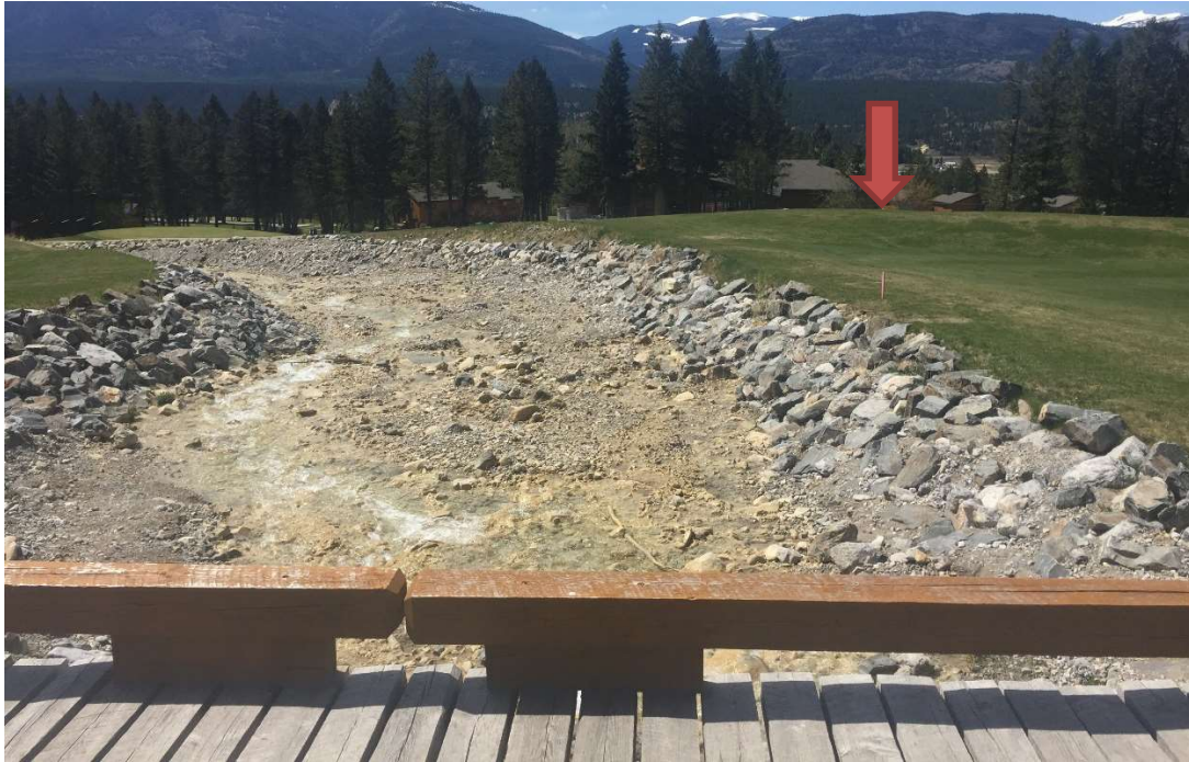
Photo 11: Golf course channel looking downstream from the cart path bridge. Channel is in good condition. The dike on the right hand side of the channel (red arrow) is in good condition. May 5, 2021.
