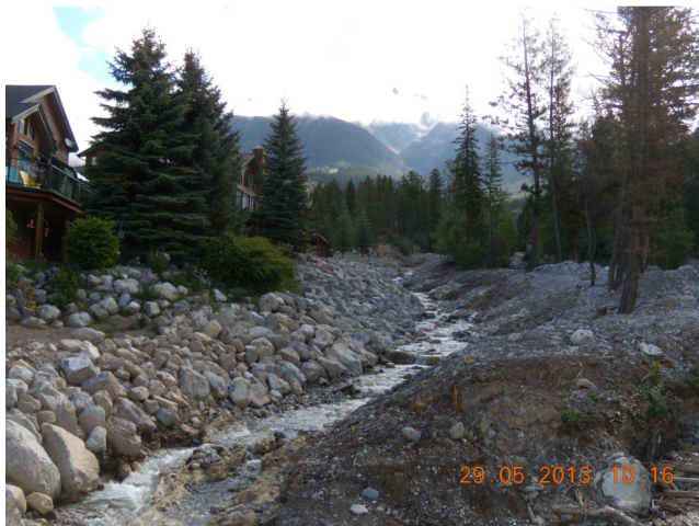
May 29, 2013 Dike/Site Conditions
