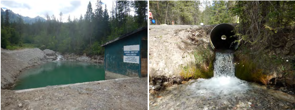
Figure 9. Fairmont Hot Springs Resort dam and irrigation reservoir within the project footprint (left), and Fairmont Resort Road crossing immediately downstream from the project (right); both are fish migration barriers.
