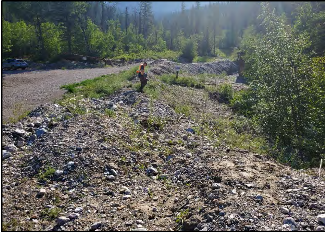
Photo 1. Existing road and evidence of flooding (view: east)
