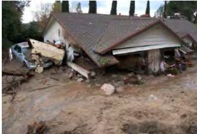
Figure 1. Downstream impacts of a post-fire debris-flow in California in 2010 (Source USGS); example of event possible at Cold Spring Creek (BGC 2020a).
