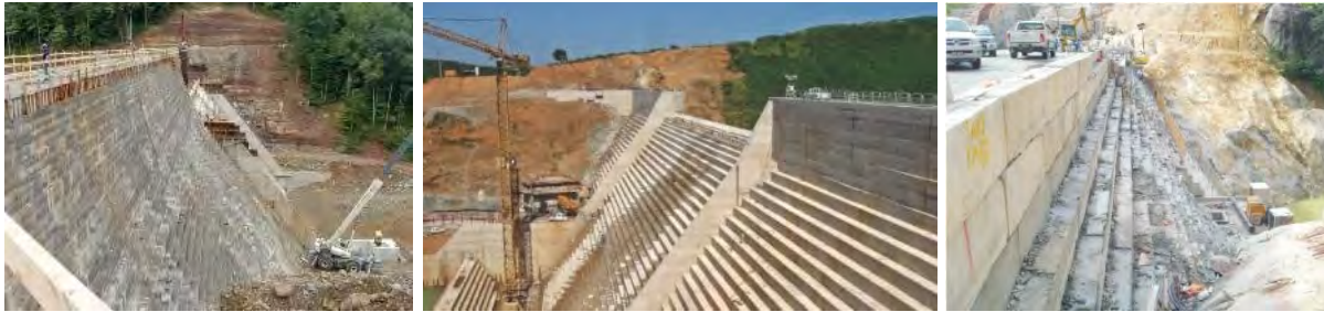
Figure 7. Examples of RCC downstream face with flat face and benching (BGC & McElhanney 2022).
