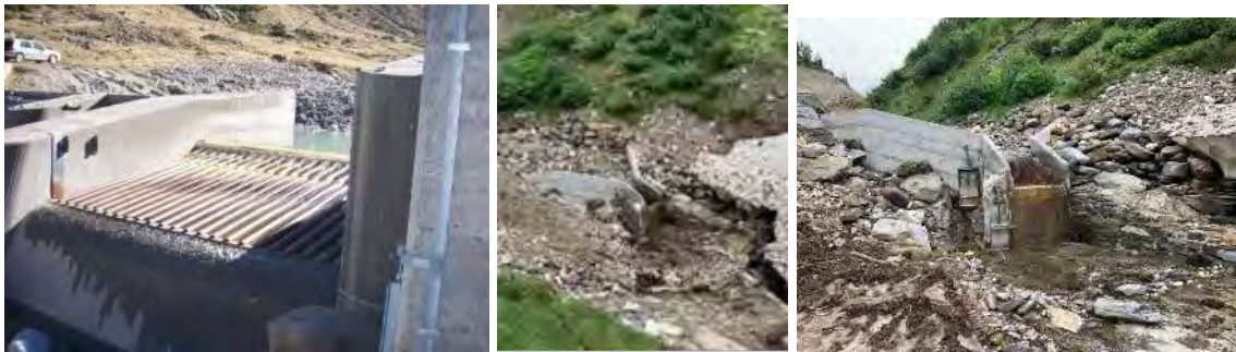
Figure 6. Tyrolean weir examples (BGC and McElhanney 2022).
