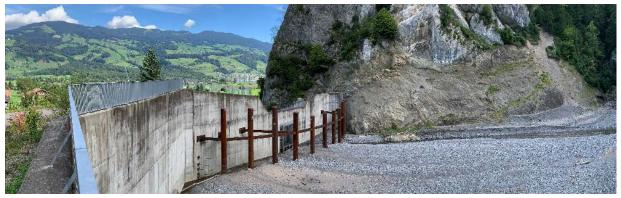
D) Filter for large woody debris (rust colored steel piles and horizontal wire ropes) upstream of an open check barrier to avoid blockage of the check barrier slot (covered with grey steel structure). Kleine Melchaa, Giswil, Switzerland (photo 2019 by M. Busslinger).
