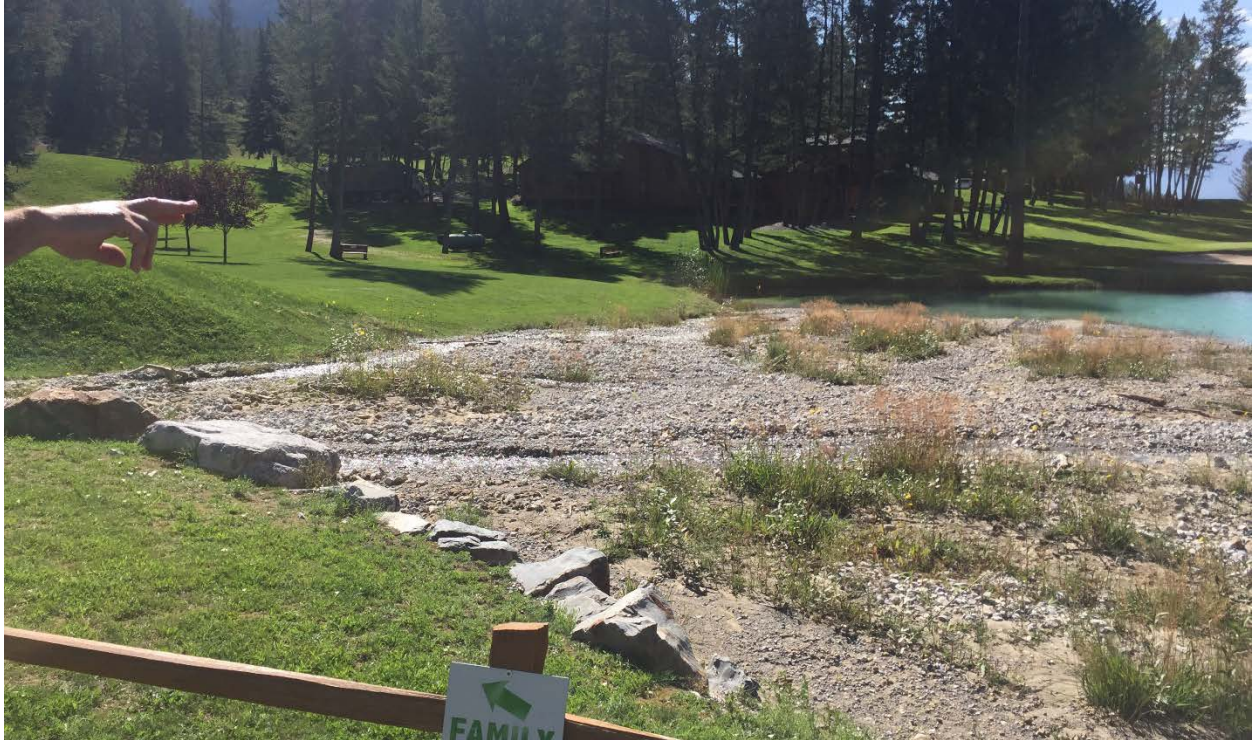
Photo 16: Entrance to the debris pond. There is a very small amount of locally eroded material recently deposited.
