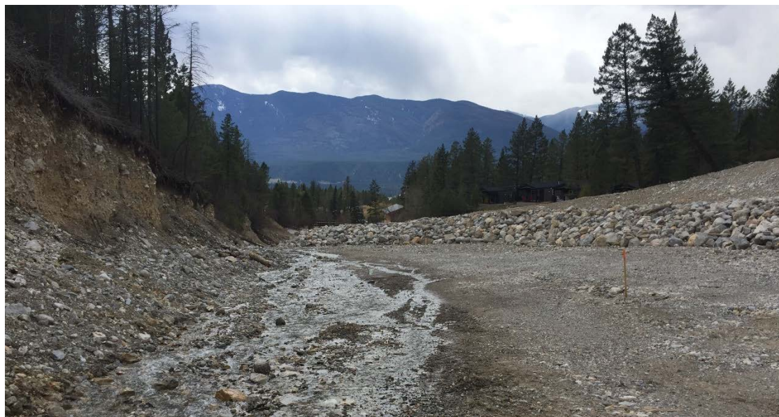
Photo 6: Bank armouring below Weir #3.
