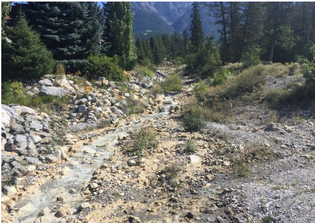
Photo 11: Looking upstream from the cart path bridge (upper extent of the Phase 1 works). No appreciable change from 2018.
