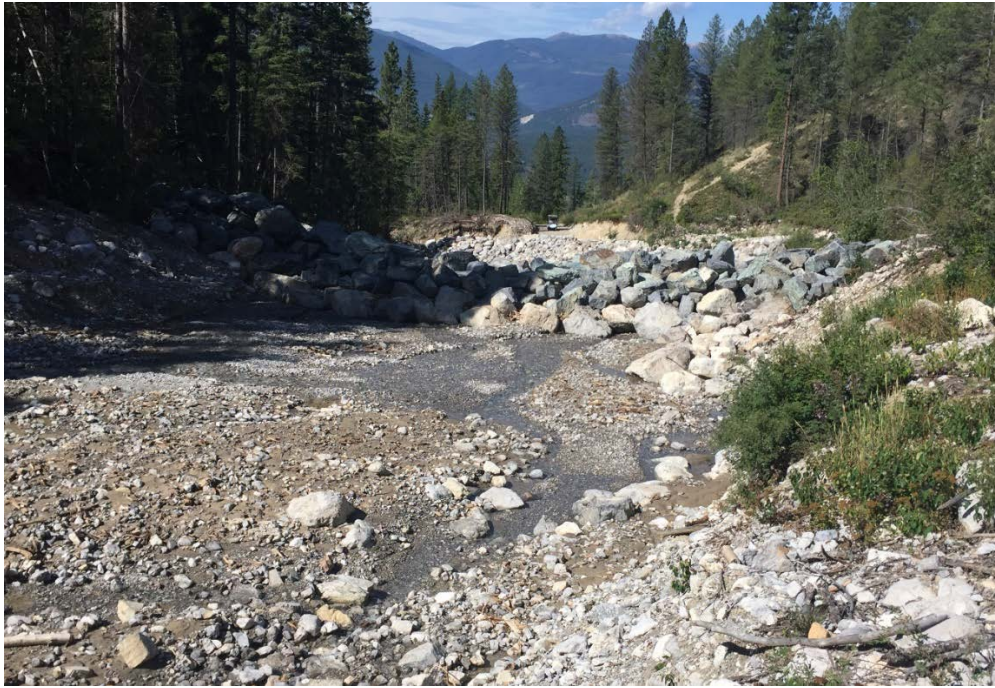
Photo 8: Weir #2, looking downstream. There is a small amount of material in front of the weir that was eroded between weirs #1 and #2.
