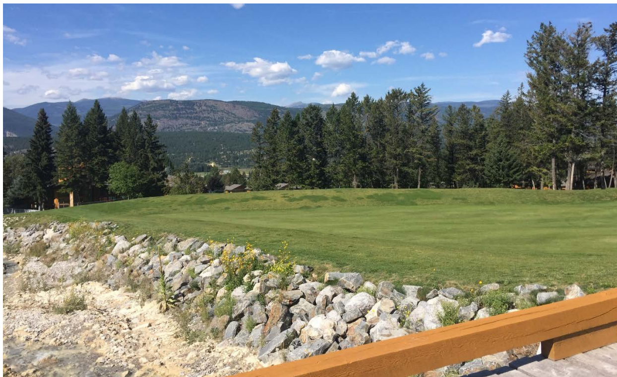
Photo 13: Right hand berm. The berm is in good condition.
