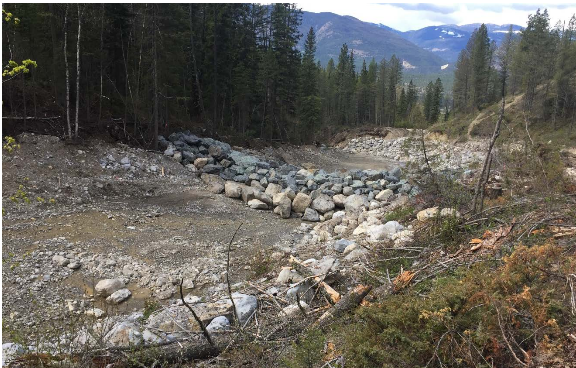
Photo 4: Weir #2 in the foreground with bank armoring in the background.
