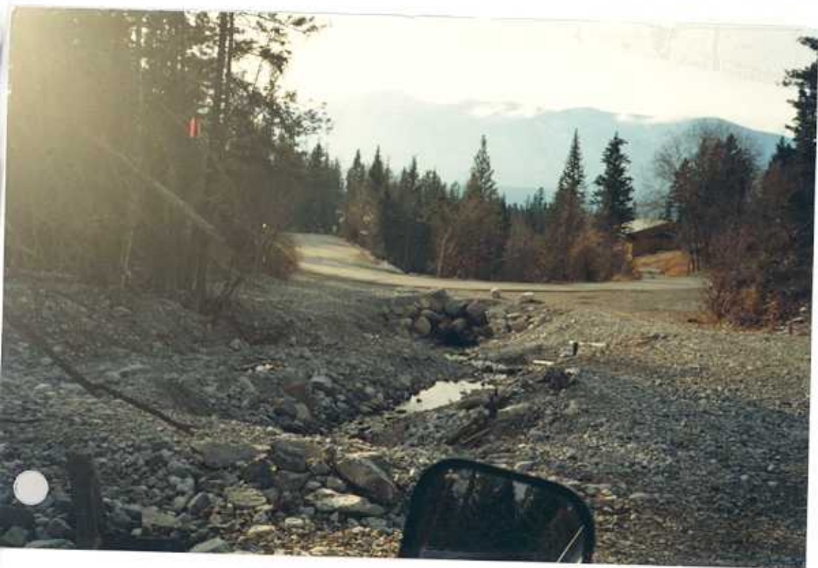
Photo #6 - Looking downstream at road crossing (see attached location map)
