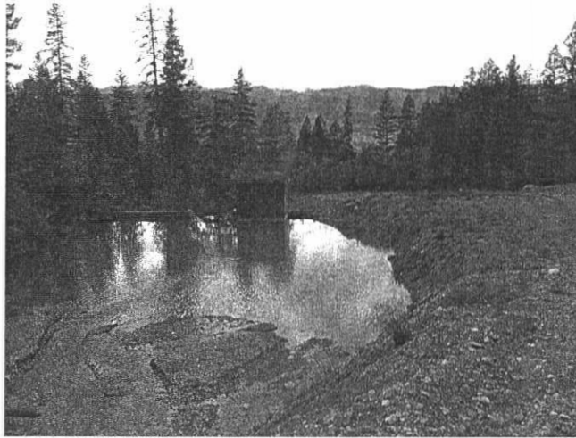
Cold Spring Creek, Site 1 - Upstream reservoir / debris trap 19/05/2005
