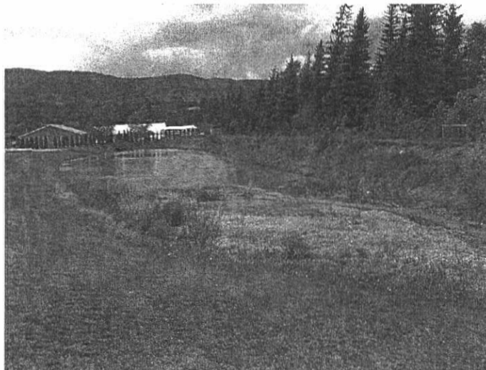
Cold Spring Creek, Site 3 – Downstream debris trap 19/05/2005
