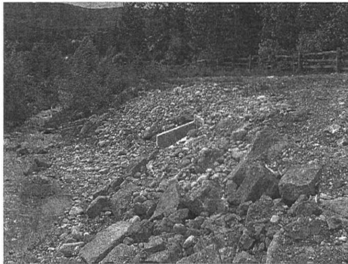
Cold Spring Creek, Site 3 – Recently constructed outfall structure 19/05/2005
