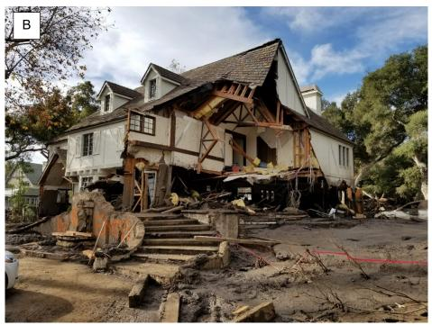
Figure 5-1. Damage by the January 9, 2018 debris flow at Montecito, California of homes impacted with an approximate impact index of > 10 m<sup>3</sup>/s<sup>2</sup>. Flow depth appears to have been approximately 2 to 3 m. Photo: Courtesy Jason Kean, United States Geological Survey.
