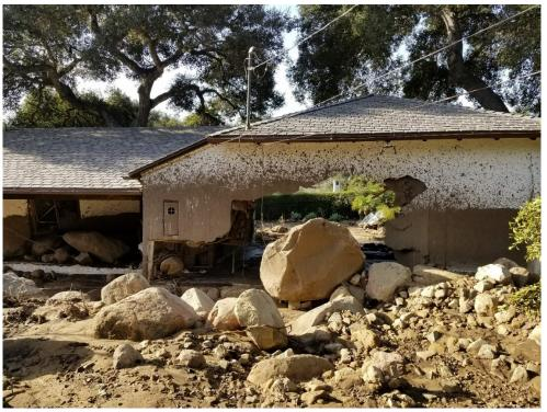
Figure 5-2. Damage by the January 9, 2018 debris flow at Montecito, California at a home impacted with an approximate impact index of 3 to 10 m<sup>3</sup>/s<sup>2</sup>. Flow depth appears to have been approximately 1.5 m. Photo: Courtesy Jason Kean, United States Geological Survey
