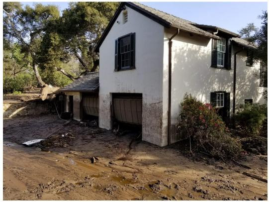
Figure 5-3. Damage by the January 9 Montecito debris flow, California at a home impacted with an approximate impact index of < 3 m<sup>3</sup>/s<sup>2</sup> and a flow depth of approximately 1.2 to 1.5 m. Image: Courtesy Jason Kean, United States Geological Survey.
