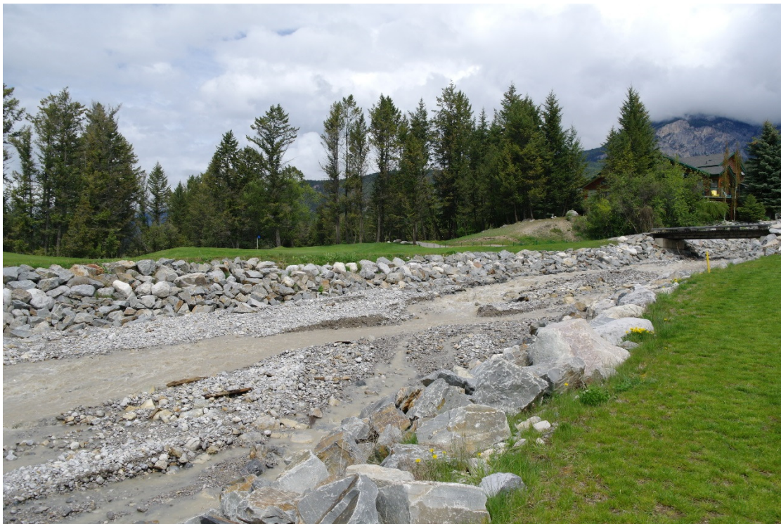
Photo 11: The widened section of creek below the cart path.
