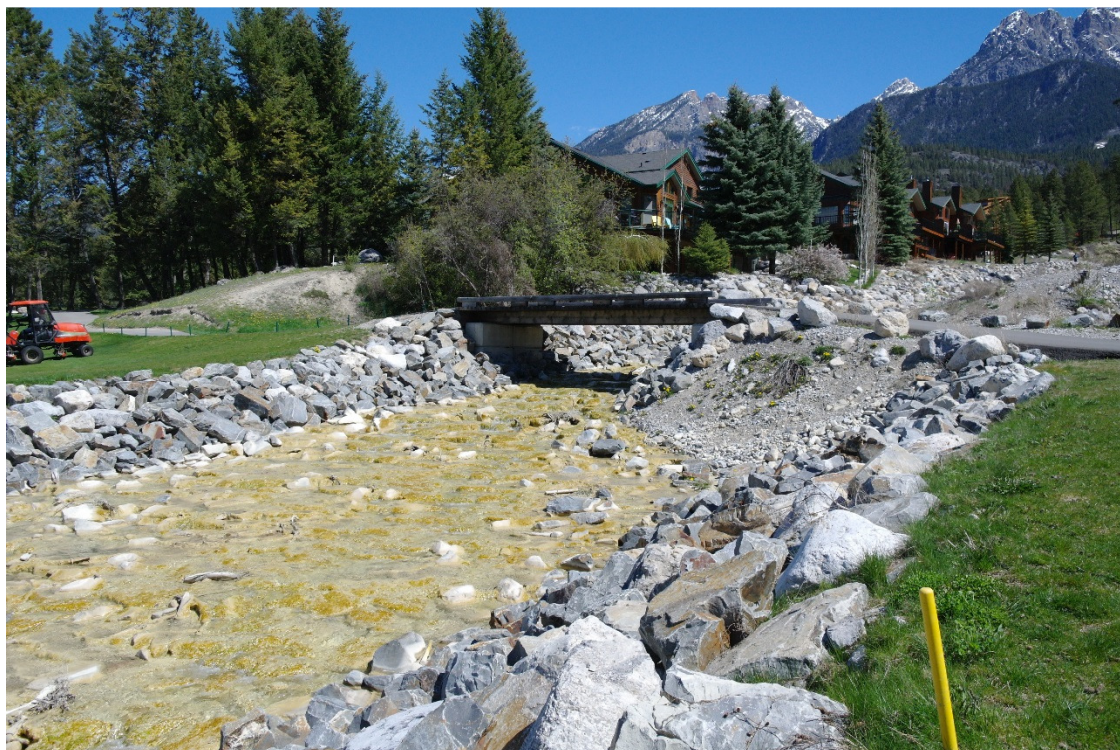
Photo 3: Cart Path Bridge at the upstream end of the golf course section of the channel.
