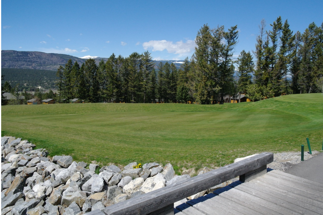
Photo 4: Right bank berm. Picture taken from the cart path bridge.
