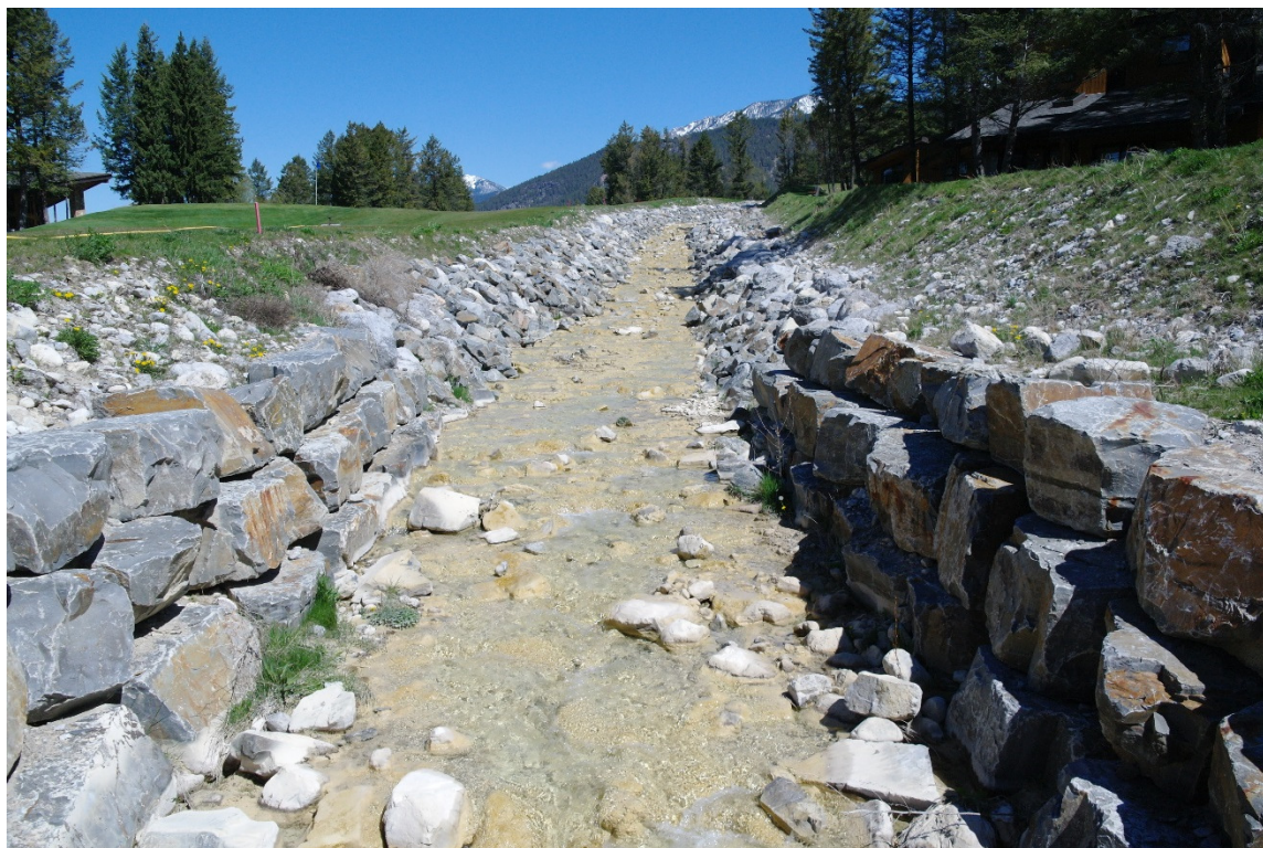
Photo 2: Looking upstream from the pedestrian bridge on the previous photo.
