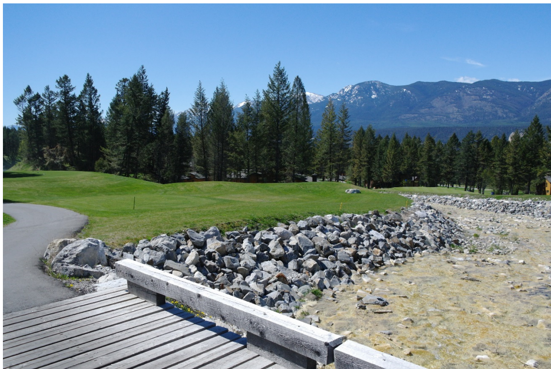
Photo 6: Left bank berm. Picture taken from the cart bridge.
