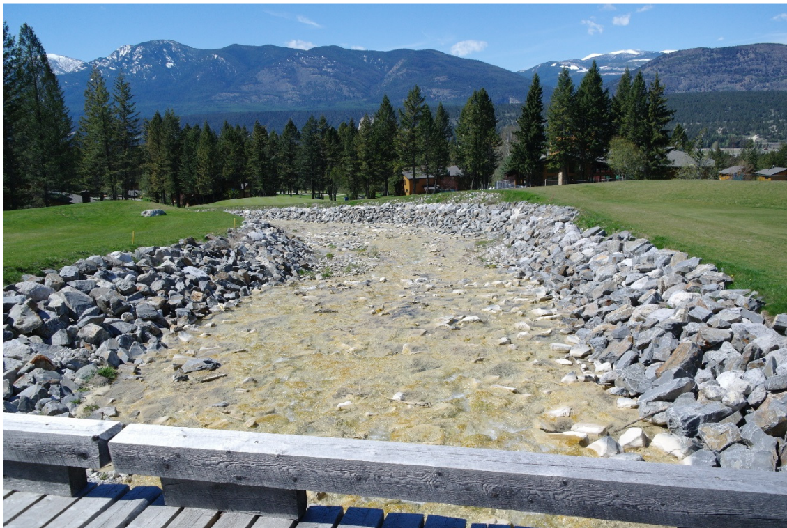
Photo 5: Widened channel. Picture taken from the cart path bridge.
