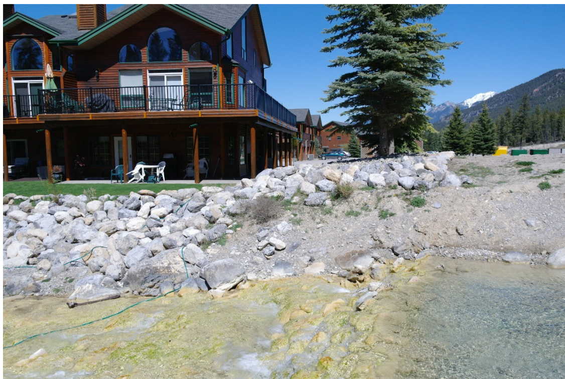
Photo 7: Upstream extent of the DFA works and bank protection.
