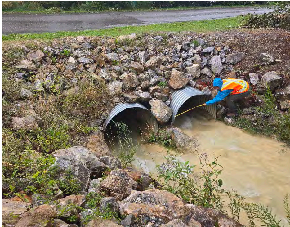
Figure A-14 Upstream end of the twinned culverts at Fairmont Creek Road. Photo taken by BGC on August 28, 2024.
