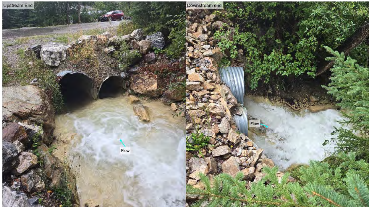
Figure A-13 Twinned culverts at Columbia River Road crossing. Photos taken by BGC on August 28, 2024.
