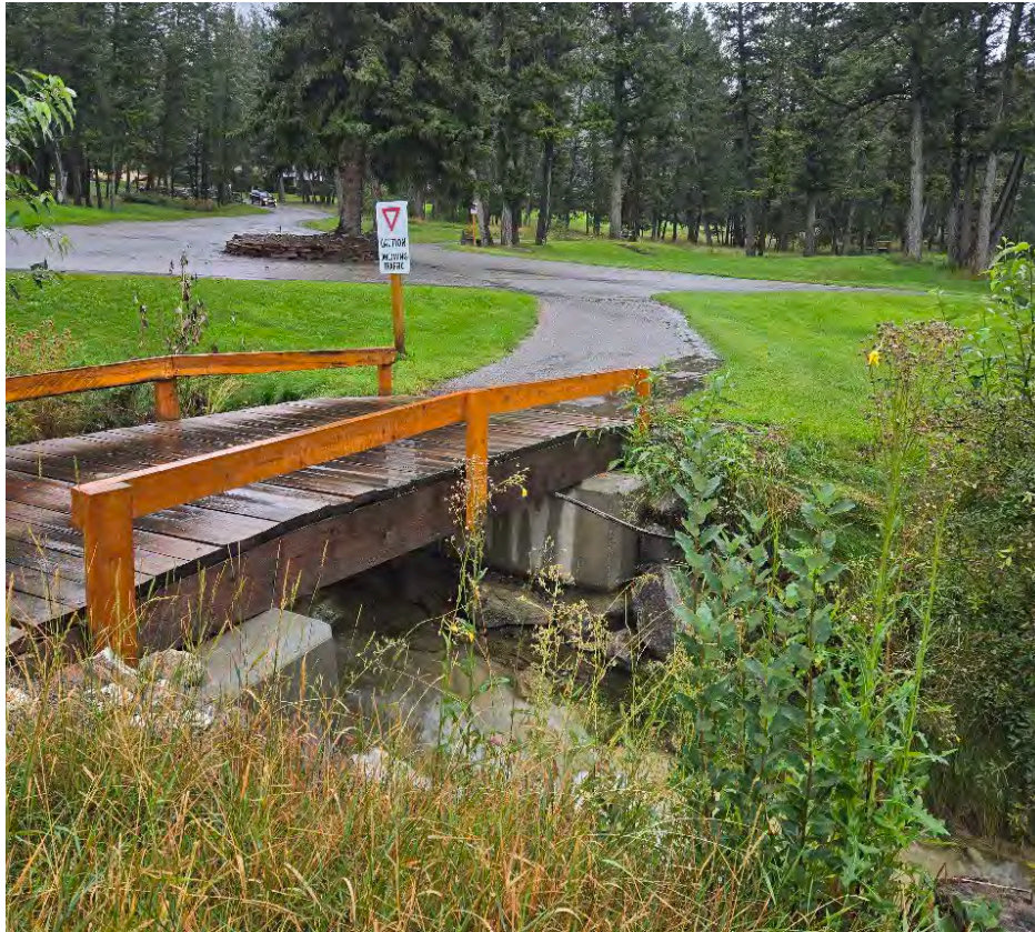
Figure A-12 Downstream end of the golf cart path bridge. Photo taken by BGC on August 28, 2024.
