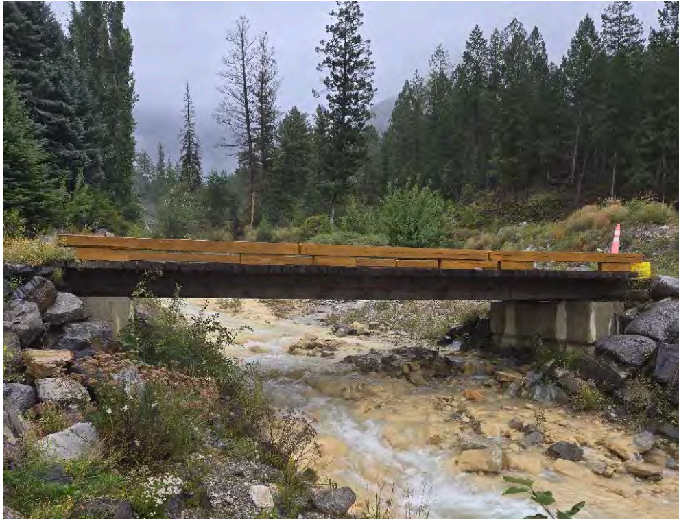
Figure A-5 Golf course bridge 1 at the downstream end of Marble Canyon. Photo taken looking upstream by BGC on August 28, 2024.
