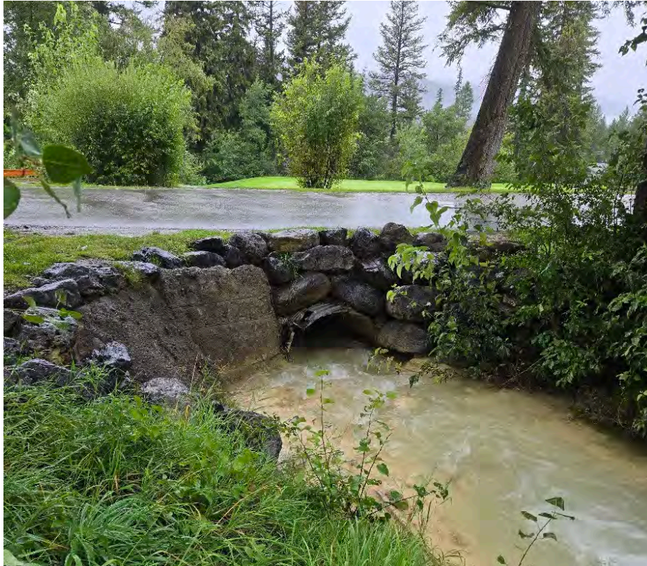
Figure A-11 Upstream view of the Mountainside Villas culvert. Photo taken by BGC on August 28, 2024.
