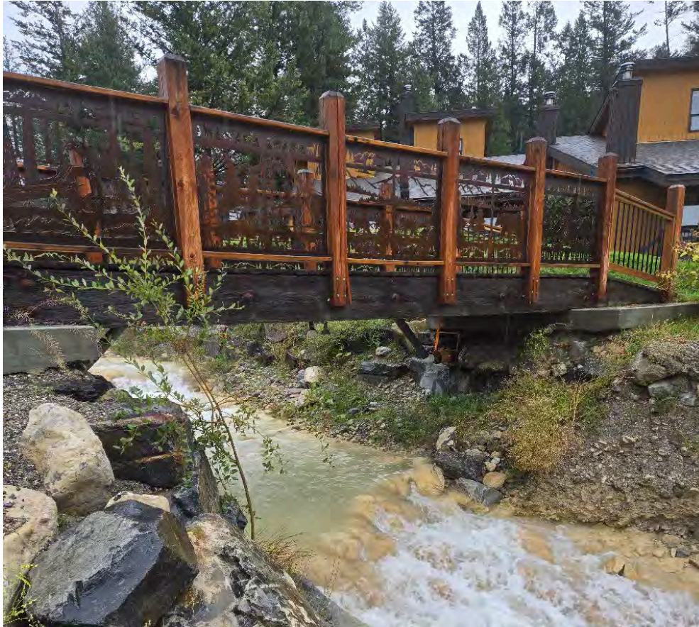
Figure A-8 Upstream view of Golf course bridge 2 at the inlet to the golf course pond. BGC photograph of August 28, 2024.
