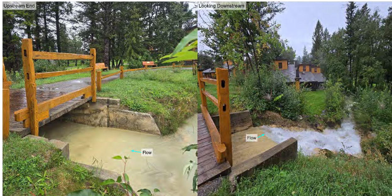
Figure A-9 Upstream and downstream views of the golf course pond outlet bridge and weir structure. BGC photographs of August 28, 2024.
