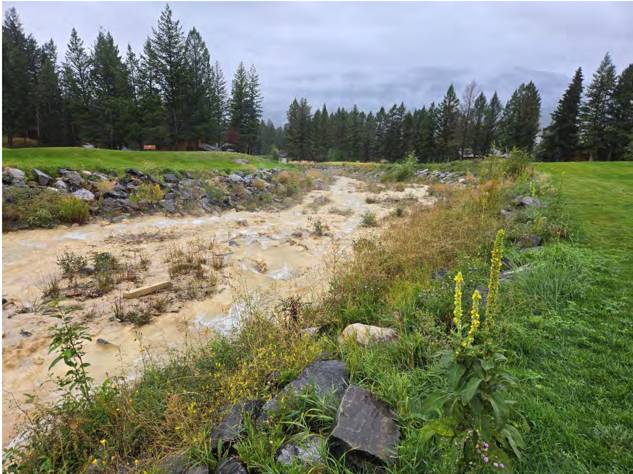
Figure A-7 Downstream view of Fairmont Creek between Marble Canyon and the golf course pond with built up and armoured banks. BGC photograph of August 28, 2024.
