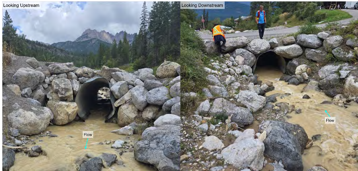
Figure A-4 Upstream and downstream views of campground access road culvert. Photos taken by BGC on August 27, 2024.
