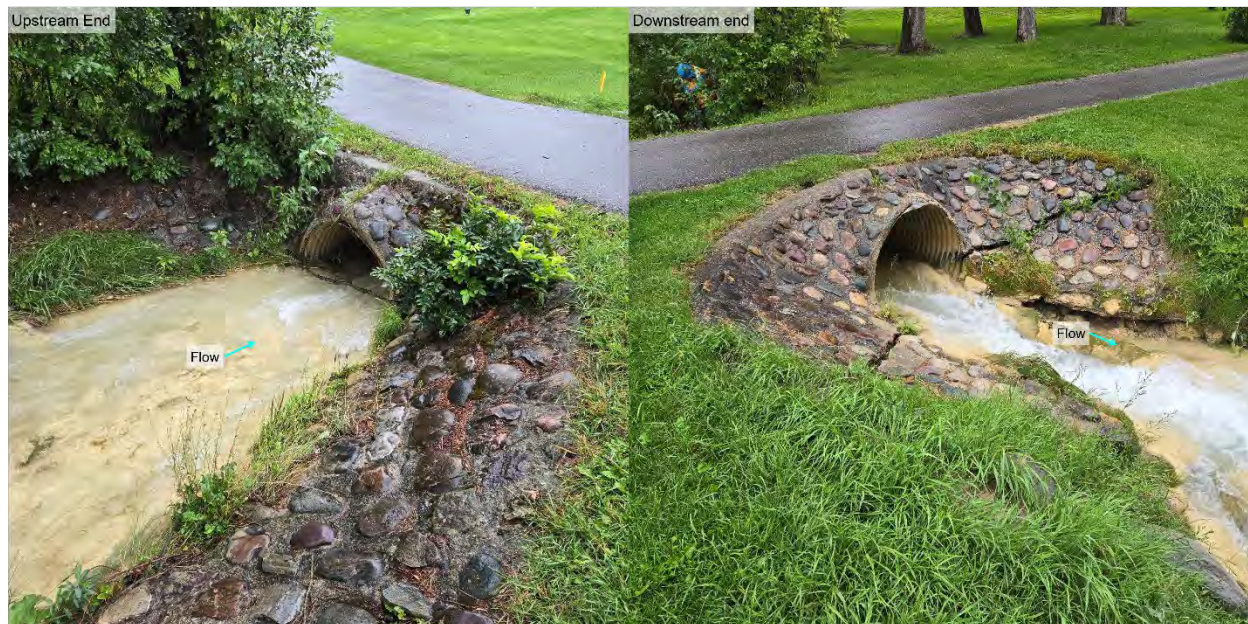
Figure A-10 Upstream and downstream views of the golf cart path culvert. Photos taken by BGC on August 28, 2024.
