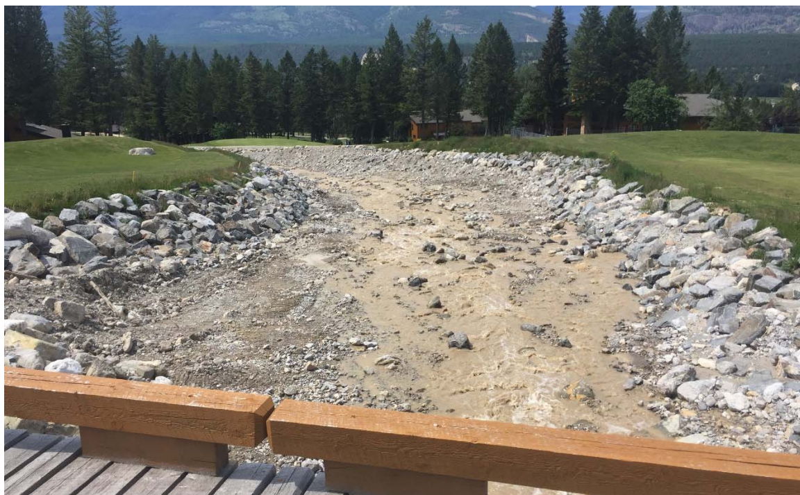
Photo 19: Golf course channel with debris material removed. June 23, 2020.
