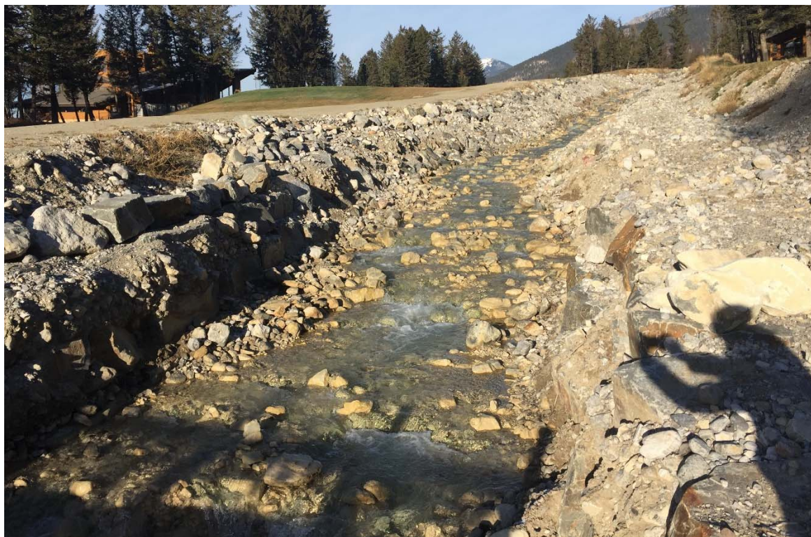
Photo 24: Lower portion of the golf course channel with debris material removed. December 4, 2020.
