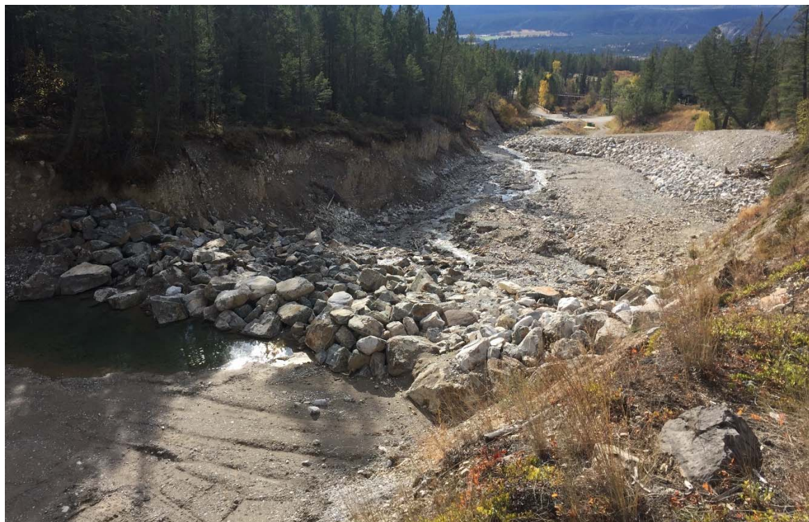
Photo 12: Weir 3 and basin after the debris material was removed. October 15, 2020.
