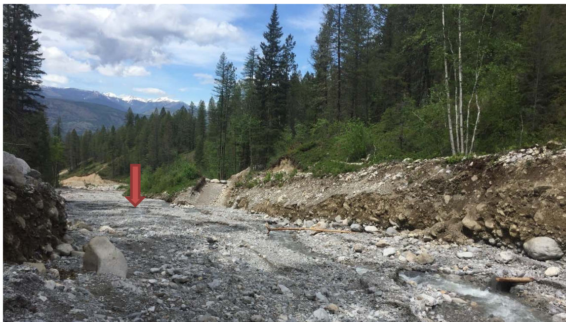
Photo 3: Weir 1 was completely covered with material from the May 31 event. The weir is located near the small access road as marked by the arrow. June 2, 2020.
