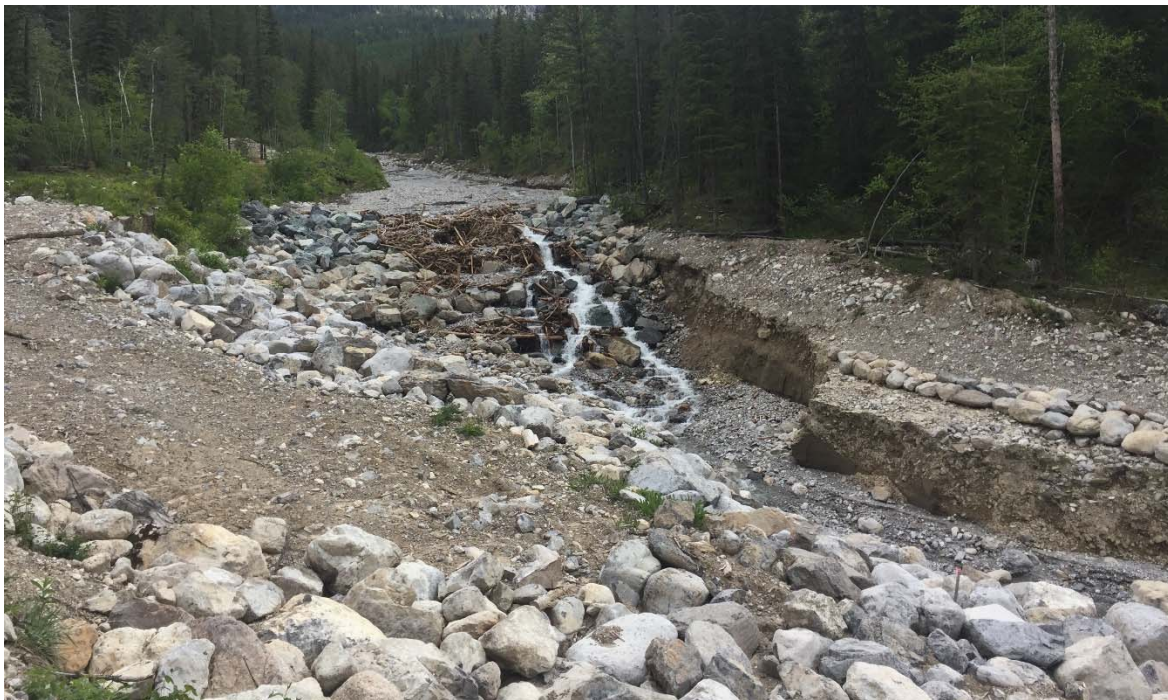
Photo 9: Weir 2 downstream face and scour after the May 31 event. This will be repaired in 2021. The armouring on the right bank was not damaged. June 4, 2020.
