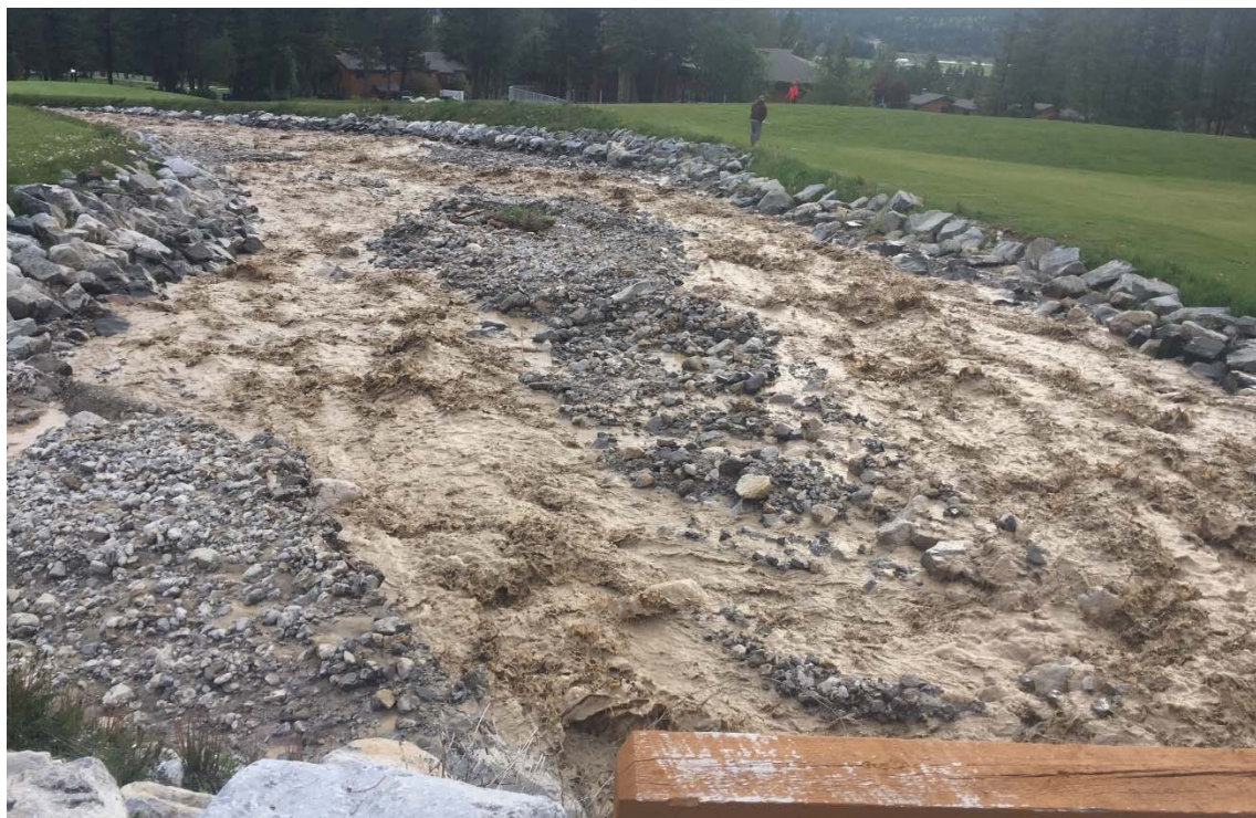
Photo 18: Golf course channel looking downstream from the cart path bridge on May 31, 2020. The debris and water were contained in the channel and the dikes were not impacted.
