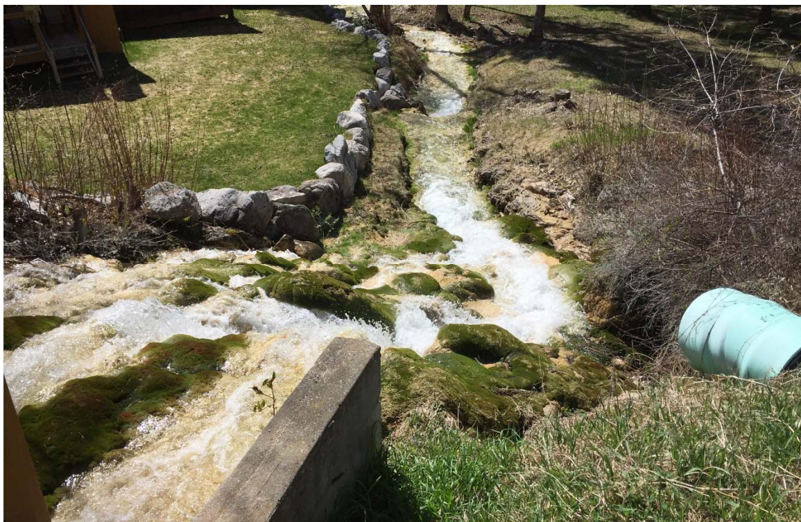
Photo 26: Pond outlet and channel in good condition. April 24, 2020.
