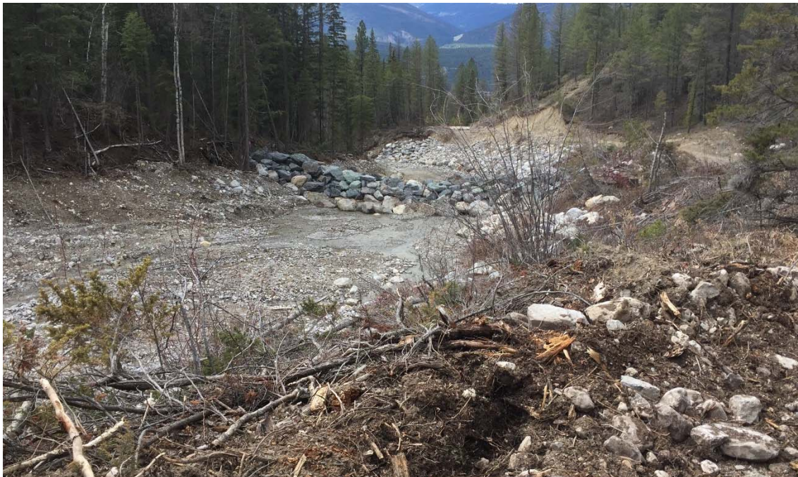
Photo 5: Weir 2 in good condition looking downstream. April 23, 2020.
