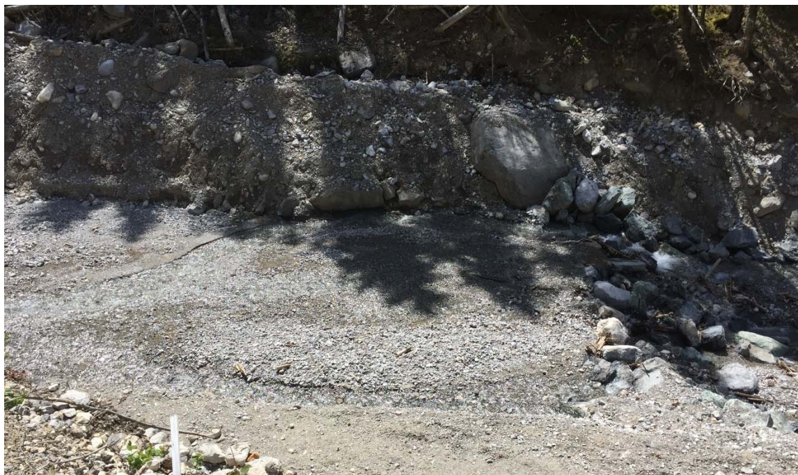
Photo 2: Weir 1, filled with debris material from the May 20 event. May 28, 2020.
