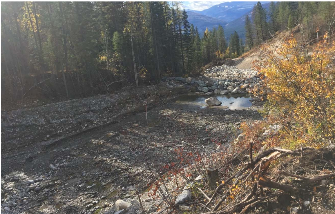
Photo 7: Weir 2 basin with debris flood material removed. October 15, 2020.
