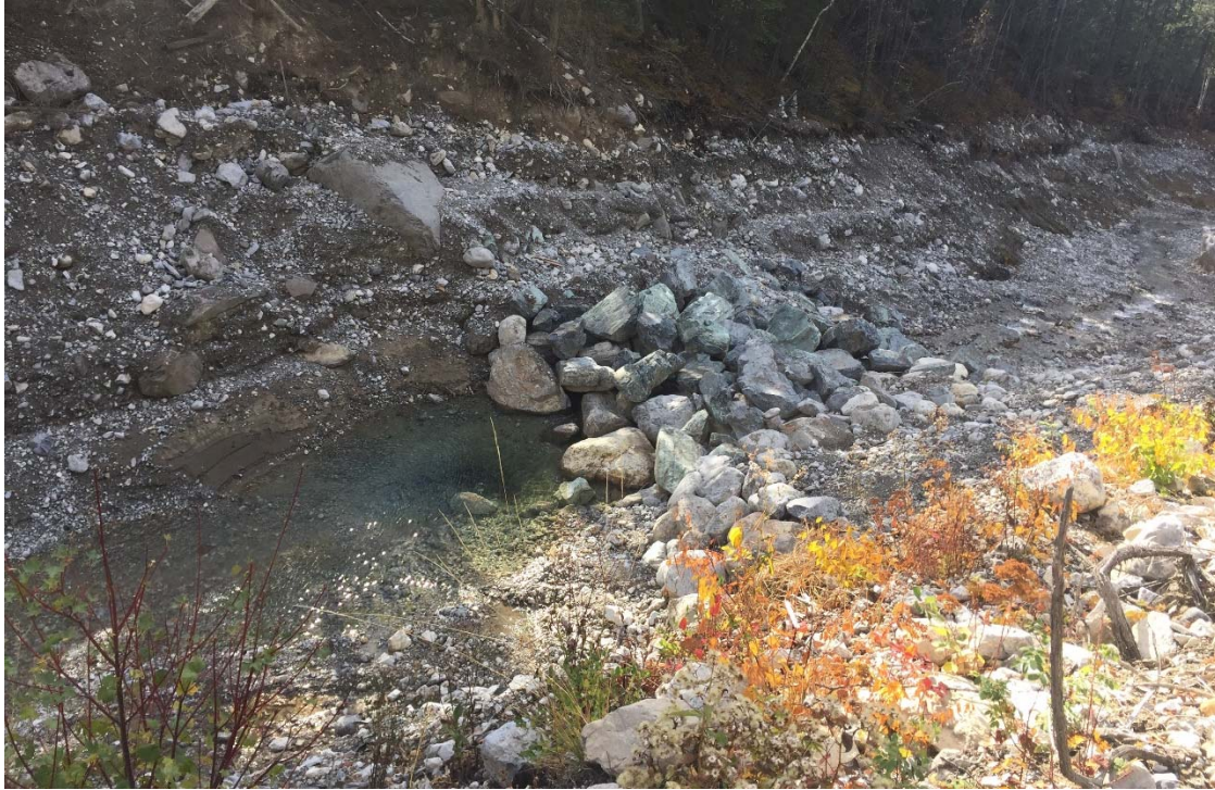
Photo 4: Weir 1 with debris flood material was removed. October 15, 2020.
