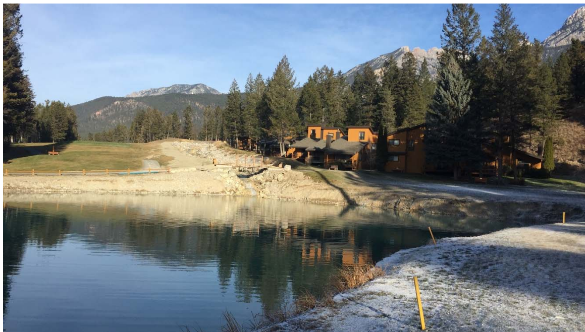
Photo 25: Hole 12 pond with debris material removed. December 4, 2020.
