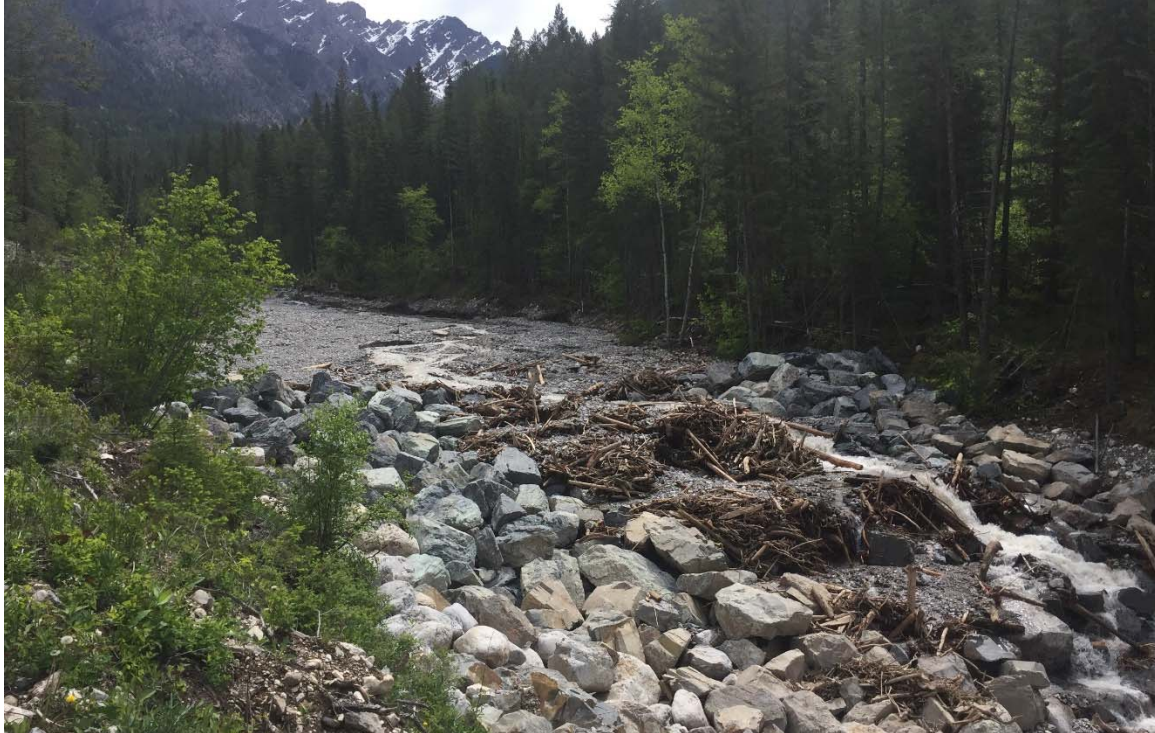
Photo 6: Weir 2 looking upstream. The basin is completely filled with debris flood material from Weir 2 continuing above Weir 1 which was buried by material. June 2, 2020.
