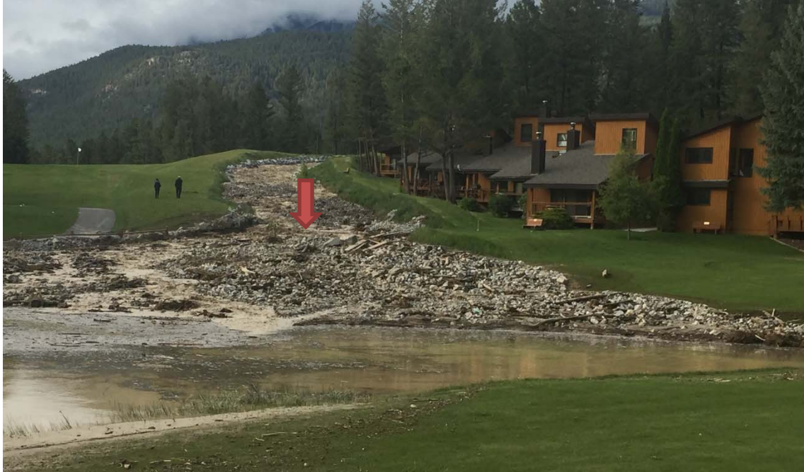
Photo 22: This photo shows the Hole 12 pond inlet and the lower channel. The lower channel was filled with debris and there was minor damage to the right hand dike. The pedestrian bridge that Photo 20 was taken from was destroyed. The pond was filled with debris. May 31, 2020.
