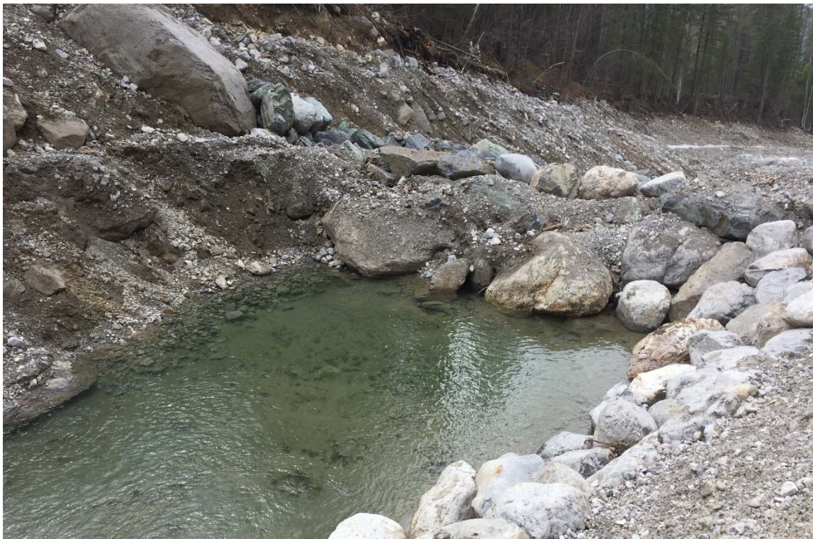
Photo 1: The uppermost weir in the system, Weir #1. April 23, 2020.
