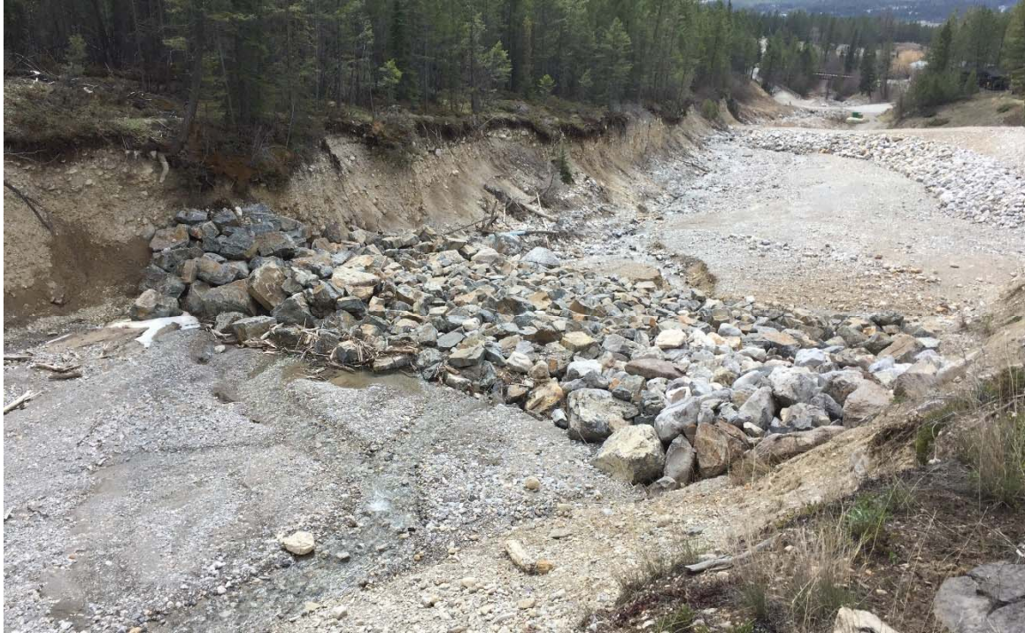
Photo 10: Weir 3 and basin in good condition. There was a very small amount of material captured behind the weir in August 2019. April 23, 2020.
