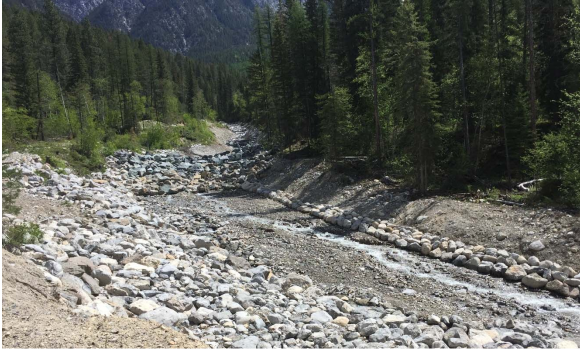
Photo 8: Weir 2 downstream face and channel in good condition. May 28, 2020.
