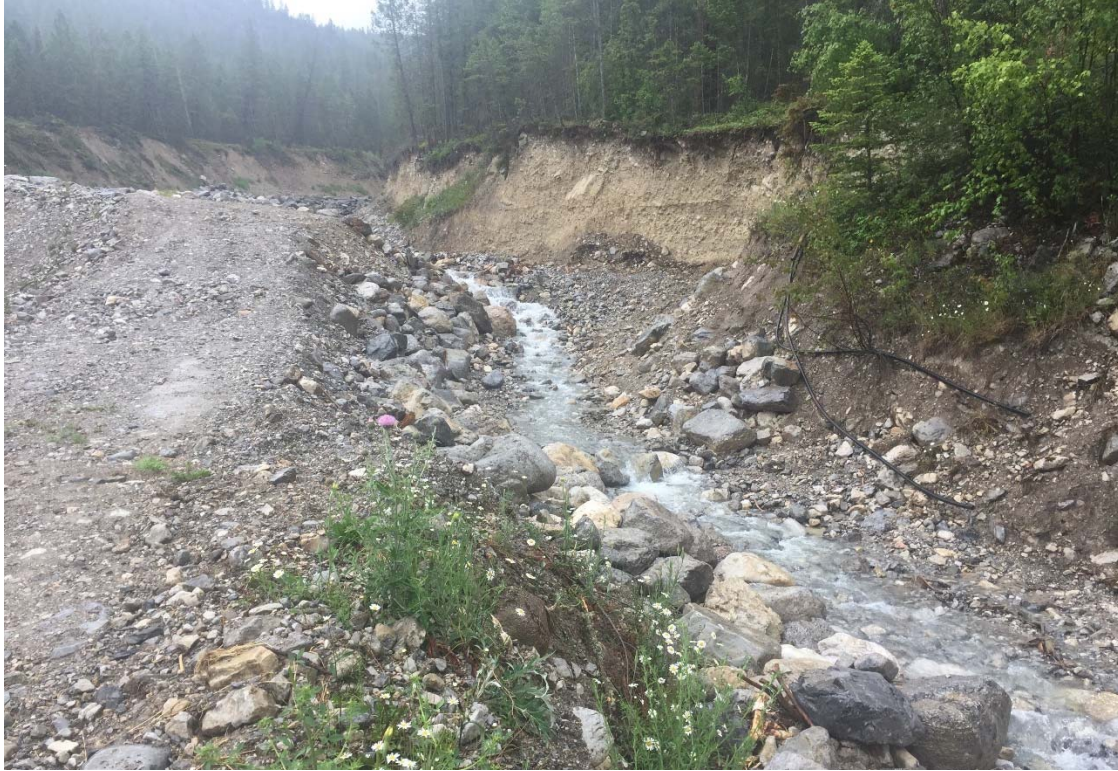
Photo 14: The berm was repaired immediately. July 7, 2020.
