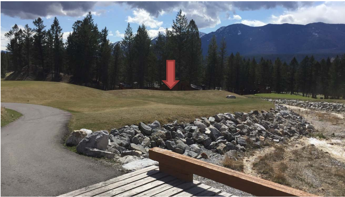
Photo 17: The left hand dike is in good condition. April 23, 2020.
