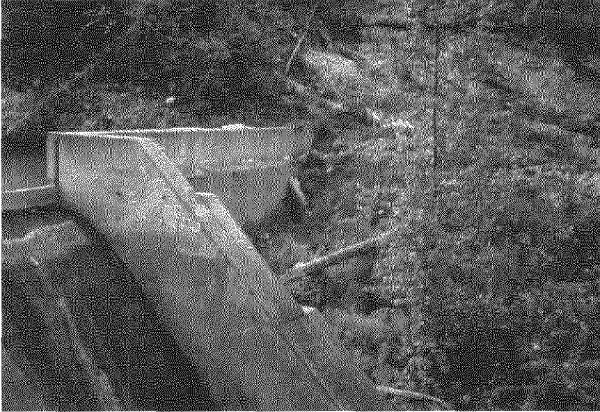
Photo 1, Coldspring Creek Dam
