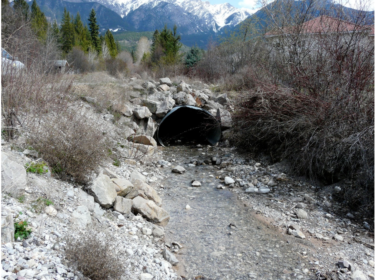
Photo 3: Lowest Cold Spring Creek culvert outlet showing gravel deposition throughout the culvert
