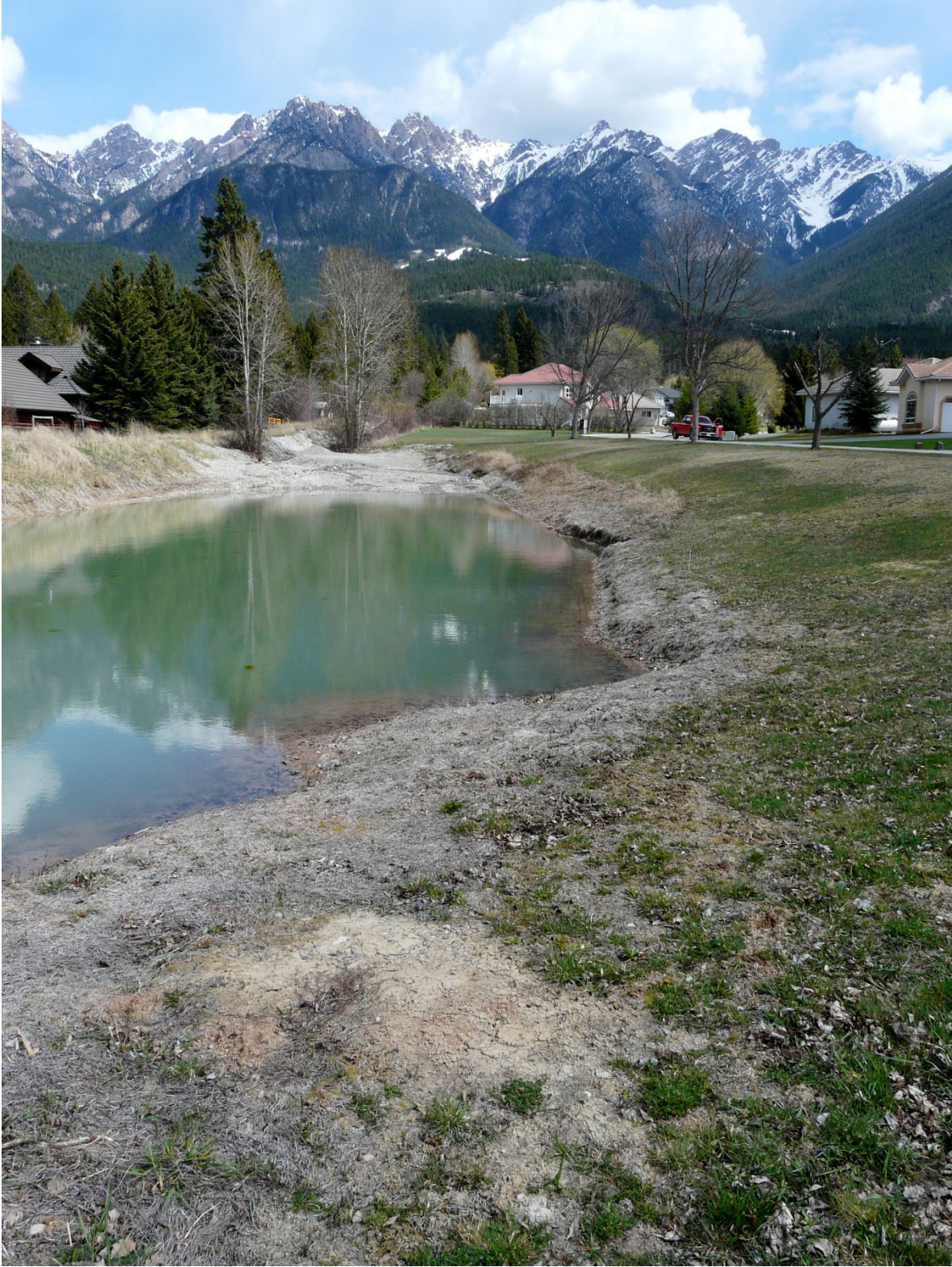
Photo 4: Cold Spring Creek debris trap showing gravel deposition at the inlet
