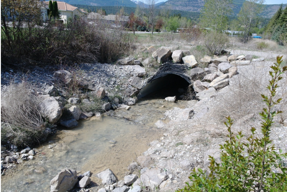
Photo 5: Inlet of the culvert above the debris pond, April 20, 2016.
