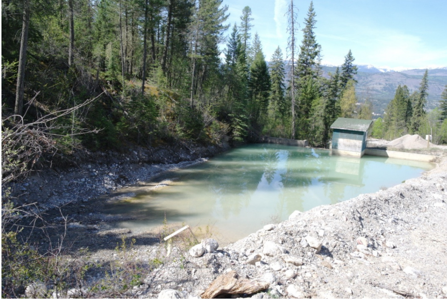
Photo 1: Cold Spring Creek Dam Reservoir, April 20, 2016. A small amount of material was removed from the reservoir by the contractor that was working just upstream of the dam.
