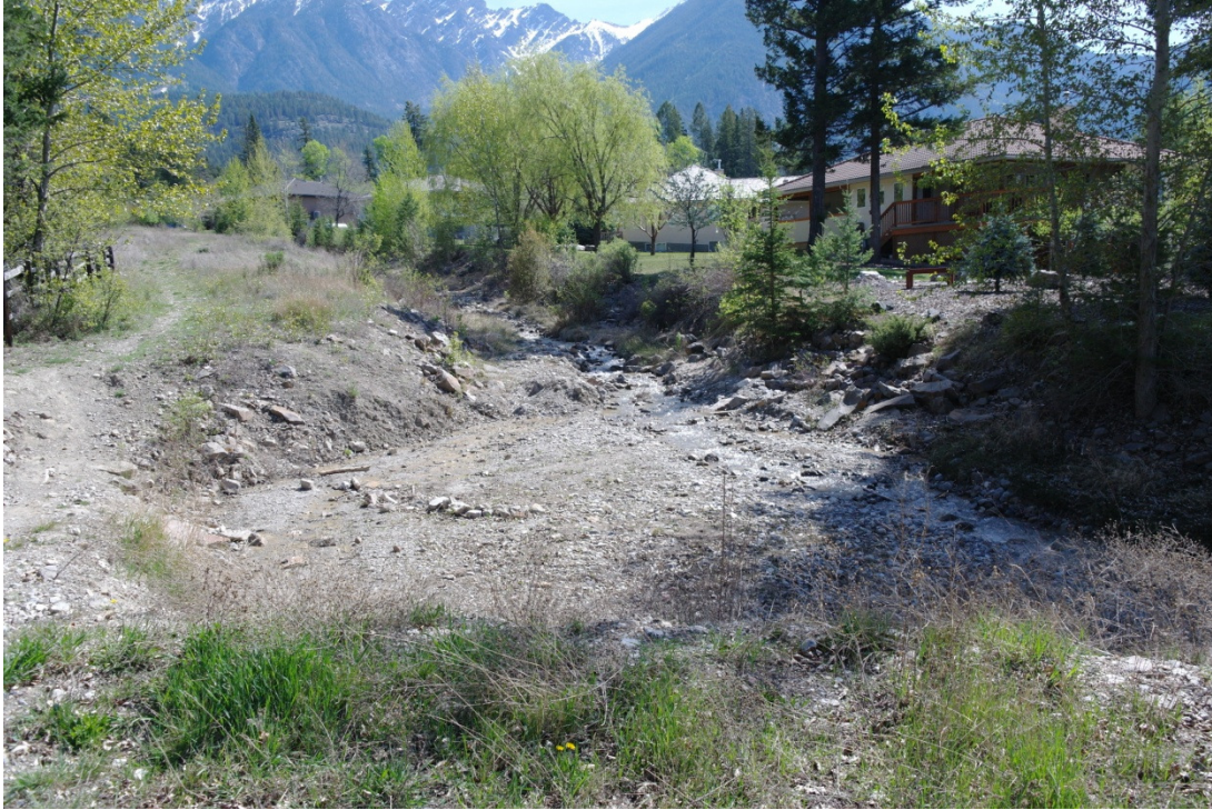
Photo 8: The mid-channel debris trap, April 20, 2016.
