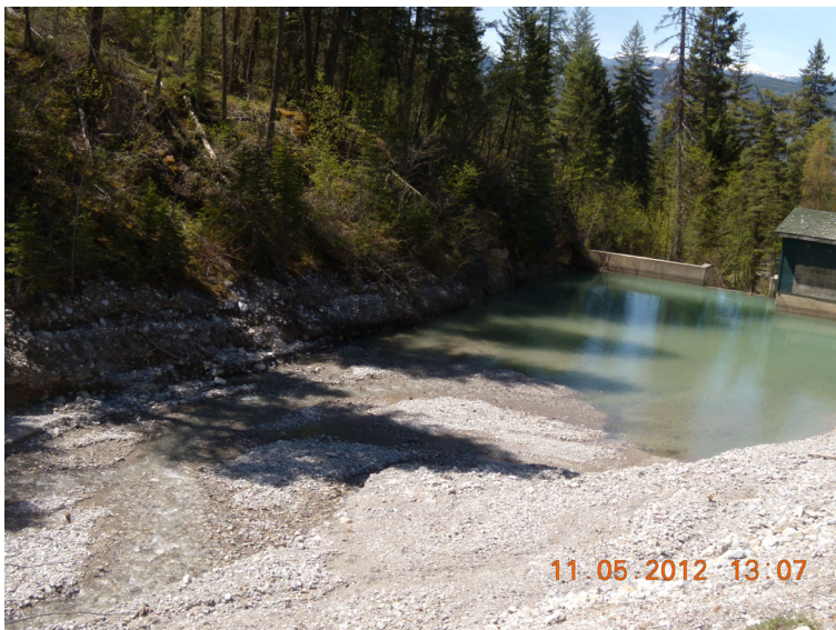
May 11, 2012 Reservoir Sediment Deposition
