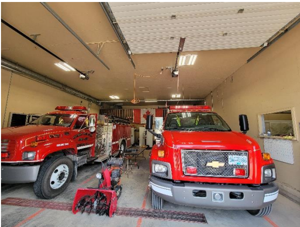
Photo 11 - Fire hall main bays in most recent addition
