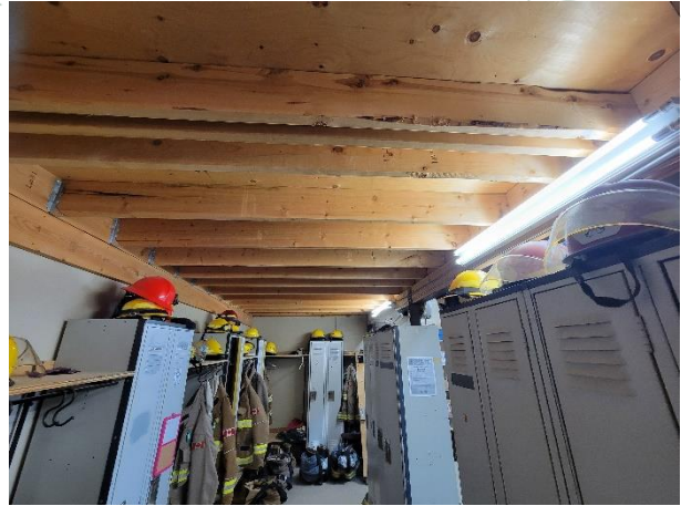
Photo 10 - Fire hall mezzanine framing
