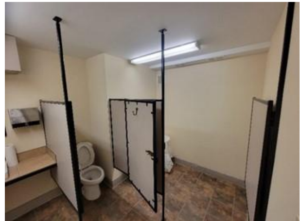
Photo 28 - Bathroom existing conditions
