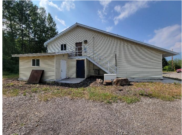
Photo 2 - Rear (north-eastern) elevation of building
