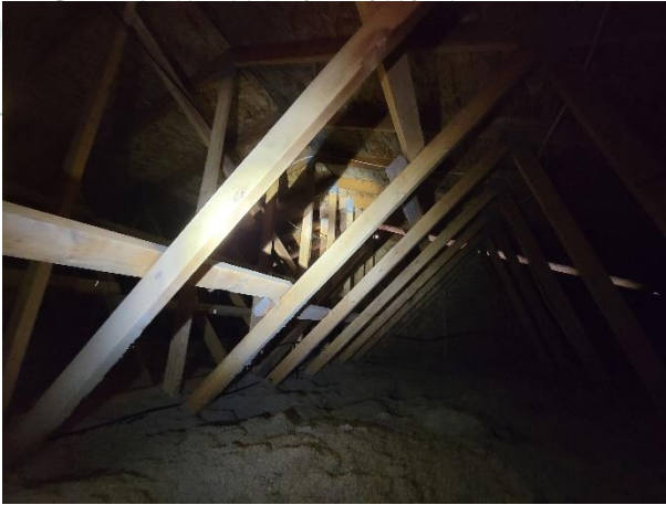
Photo 21 - Modified queenpost trusses over fire hall addition
