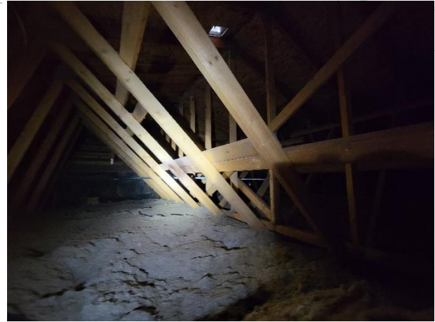
Photo 22 - Modified queenpost trusses over fire hall addition
