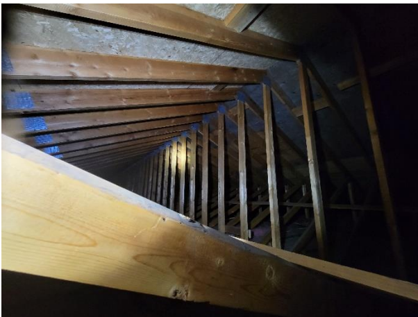
Photo 23 - Howe trusses over the original community hall building
