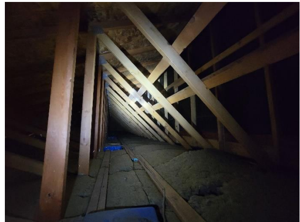
Photo 20 - Monoslope trusses over community hall addition
