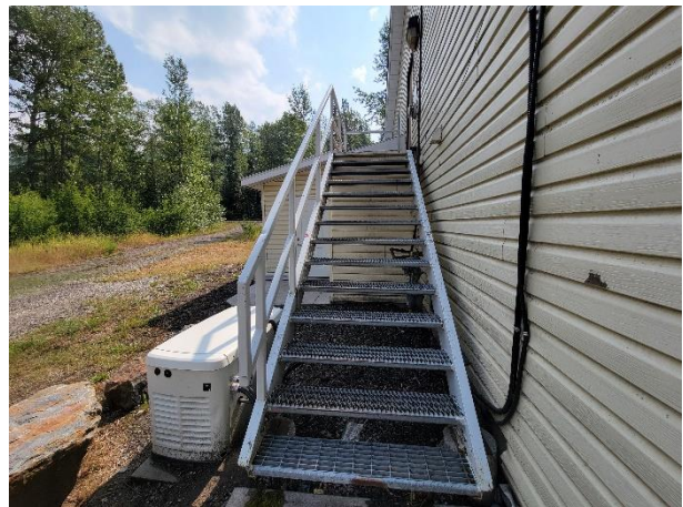
Photo 8 - Rear entry stairs
