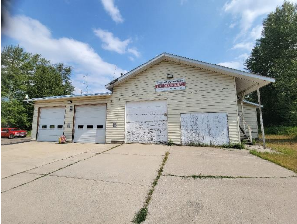
Photo 1 - Front (south-western) elevation of building
