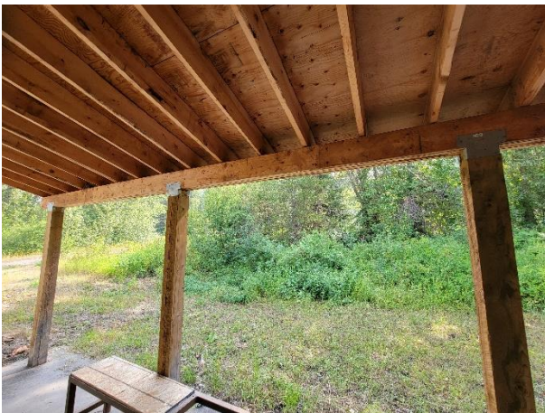
Photo 7 - North-eastern patio beam and post framing
