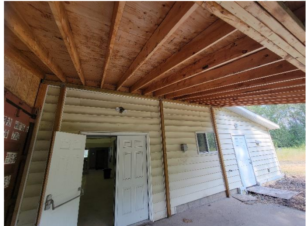
Photo 6 - North-eastern patio roof framing
