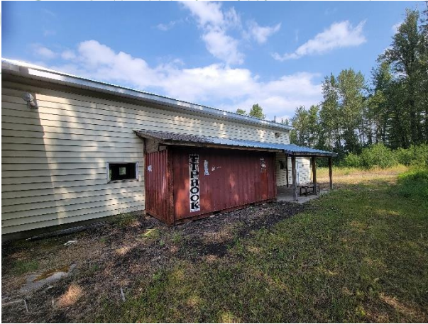
Photo 5 - Attached sea-can and patio at north-eastern corner of building
