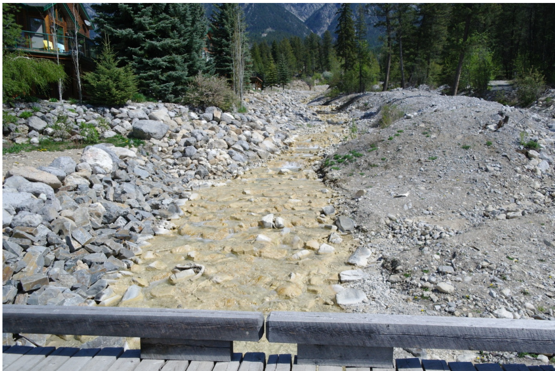
Photo 6: Left bank berm and widened channel. Picture taken from the cart path bridge.
