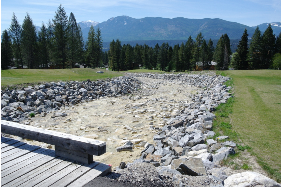
Photo 6: Left bank berm and widened channel. Picture taken from the cart path bridge.
