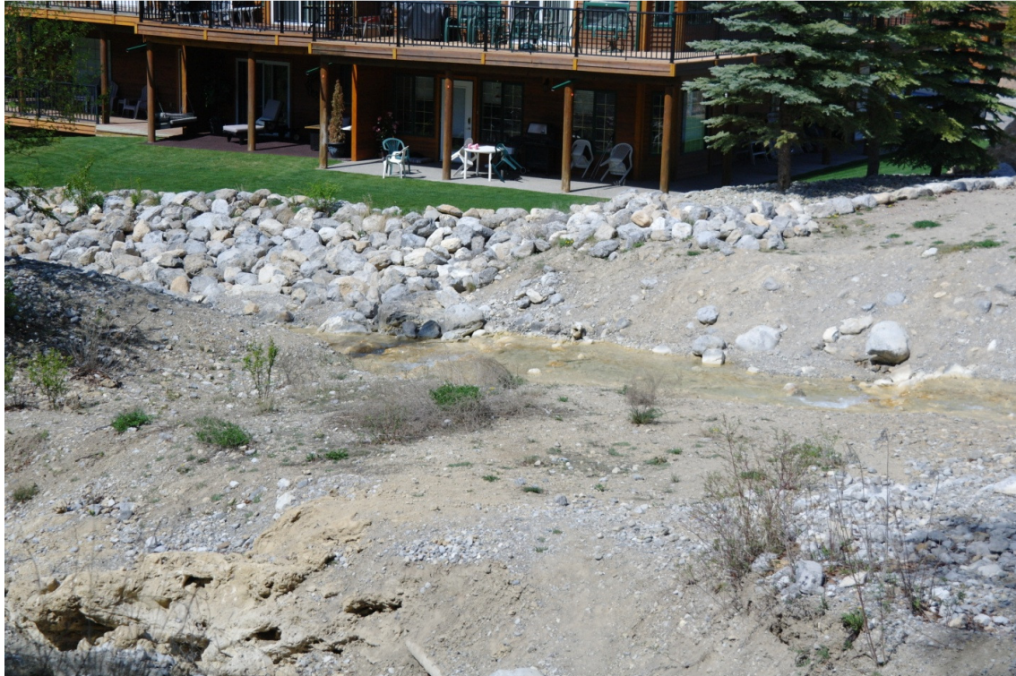
Photo 8: Upstream extent of the DFA works and bank protection.
