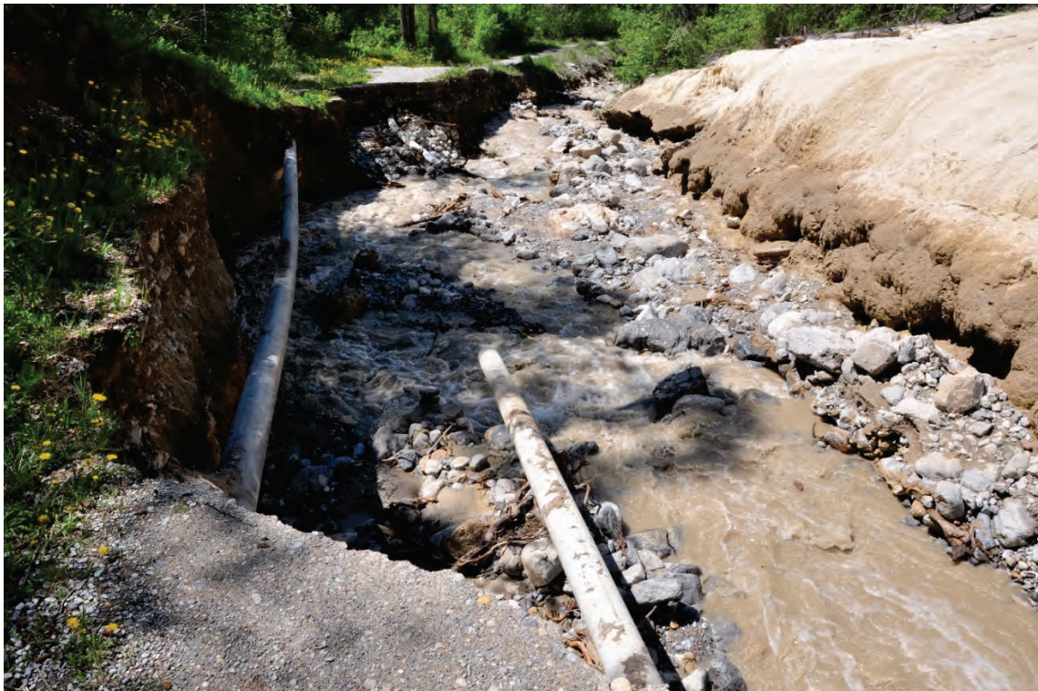
Photo 6.10 One of two extended suspended section of golf course irrigation waterline.
