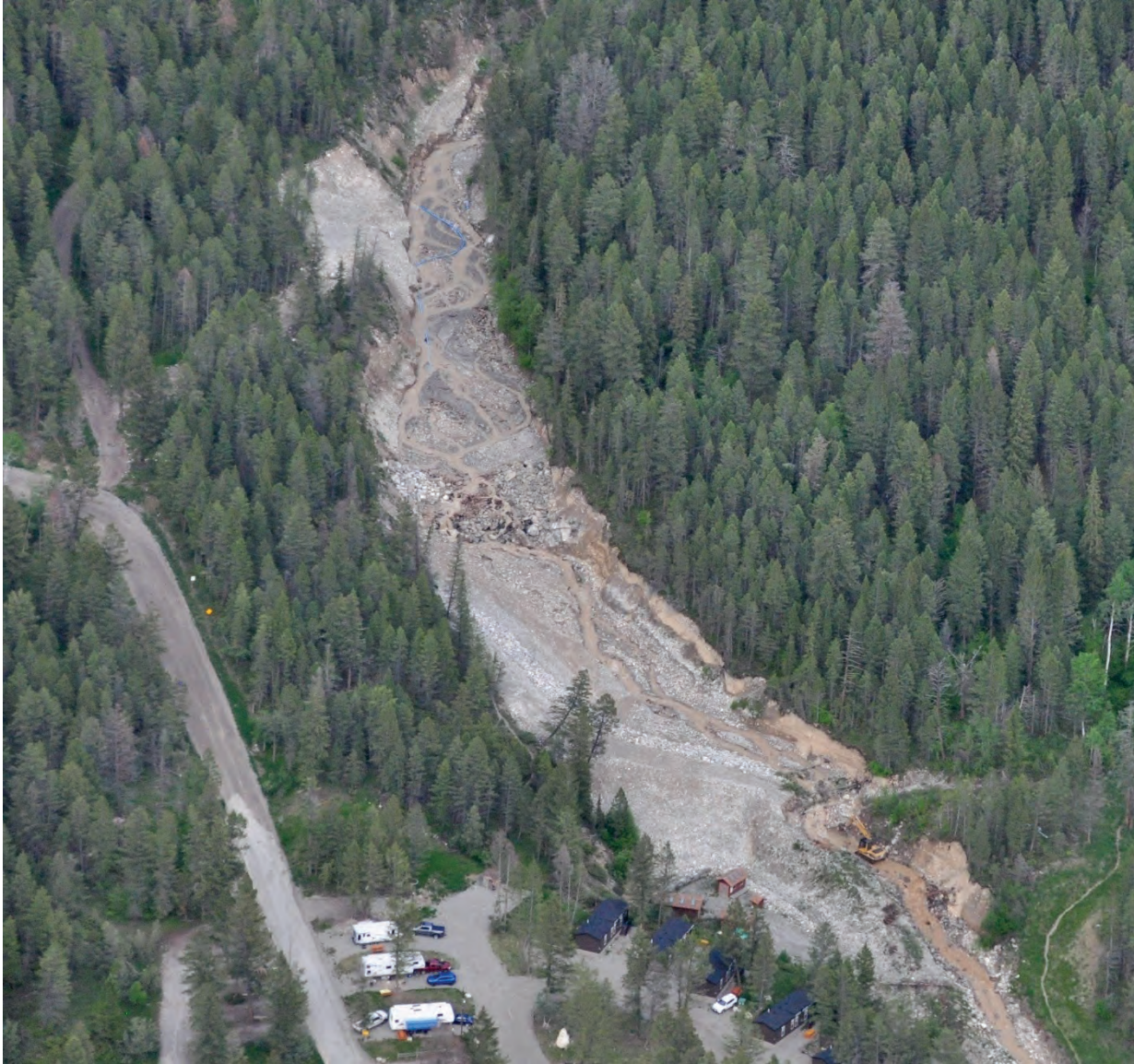
Photo 3.22 June 1 2020 helicopter photo of containment weir # 3 filled with sediment as well as degraded channel adjacent to hot spring intake buildings. The excavator working in the channel had just started to access the channel and repair the eroded bank upstream and to the left of where it is positioned in the image.
