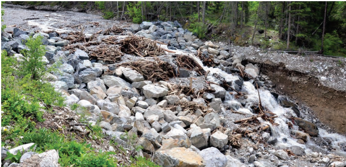
Photo 3.15 Sediment and debris that overtopped weir # 2 during the May 31, 2020 event.
