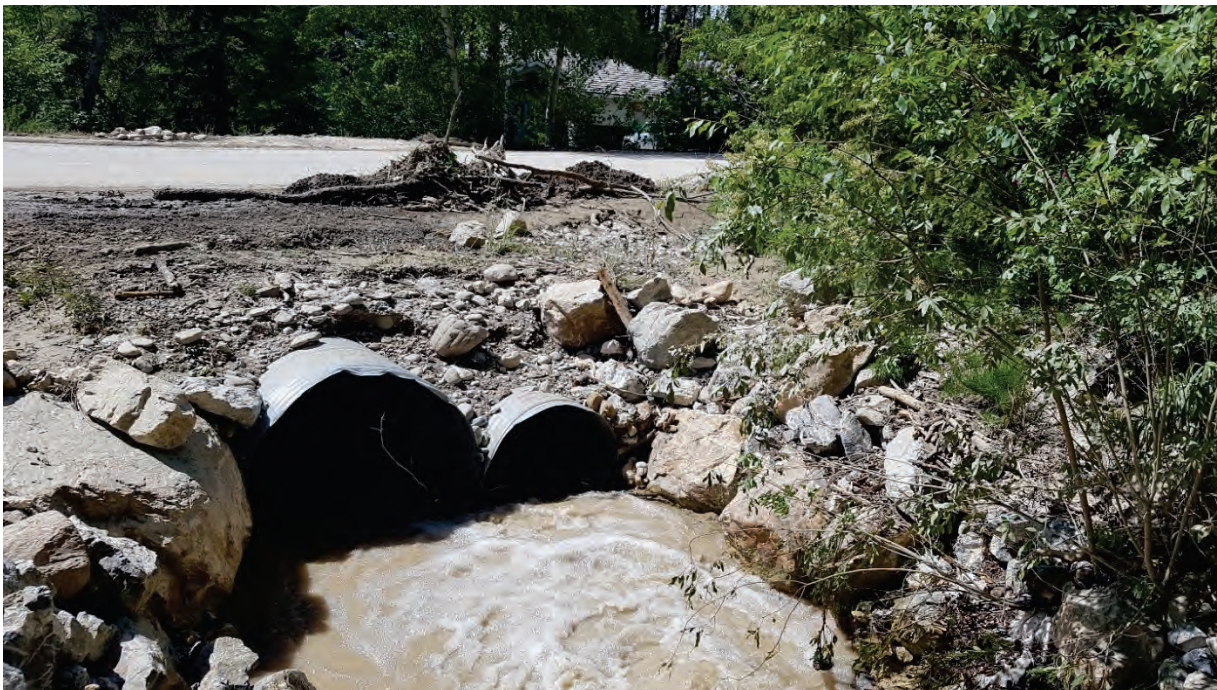
Photo 2.2 Columbia River Road crossing on Fairmont Creek that was overtopped during flood event.
