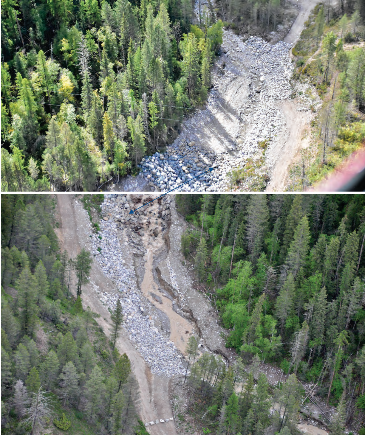
Photo 3.16 Top photo indicates the area downstream of the second debris containment weir in 2019, viewed looking downstream. The bottom photo shows the same area after then 2020 event looking upstream. The arrow links the common weir.
