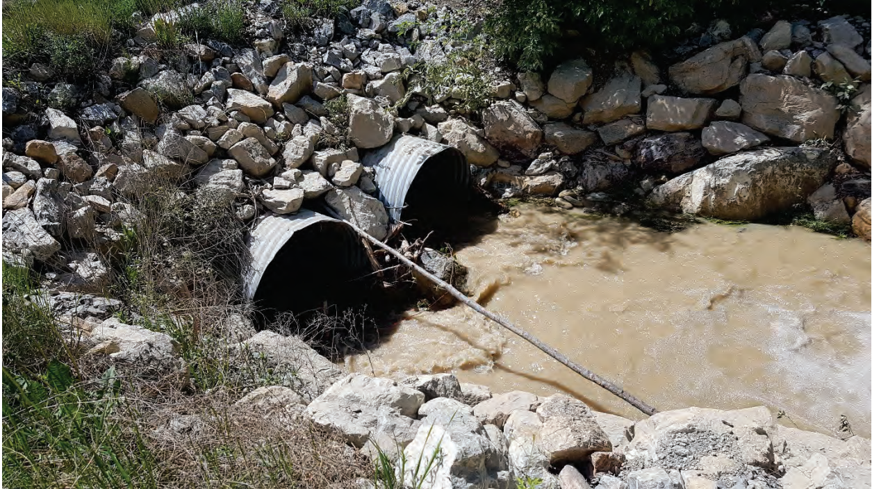
Photo 2.3 Fairmont Creek Road culvert on Fairmont Creek. This road crossing was not overtopped and a debris line can be seen about 0.3 m above the culvert.
