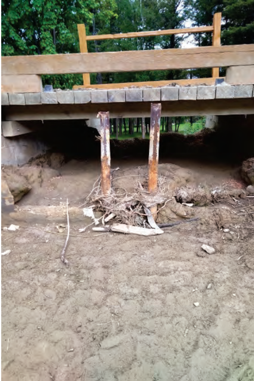
Photo 6.4 Upstream end of channel leaving golf course pond following May 2020 flood event. Photo provided by contractor excavating sediment.
