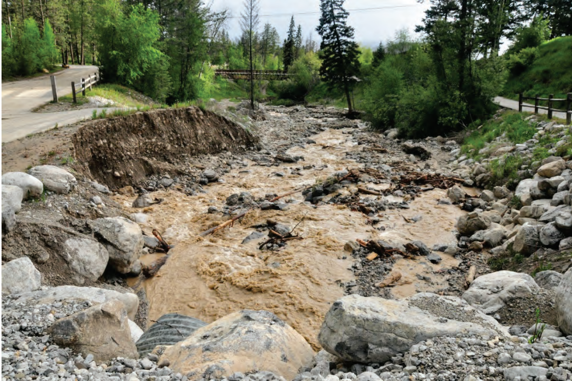
Photo 6.7 Middle portion of Fairmont Creek that would benefit from both bank protection and grade control structures.
