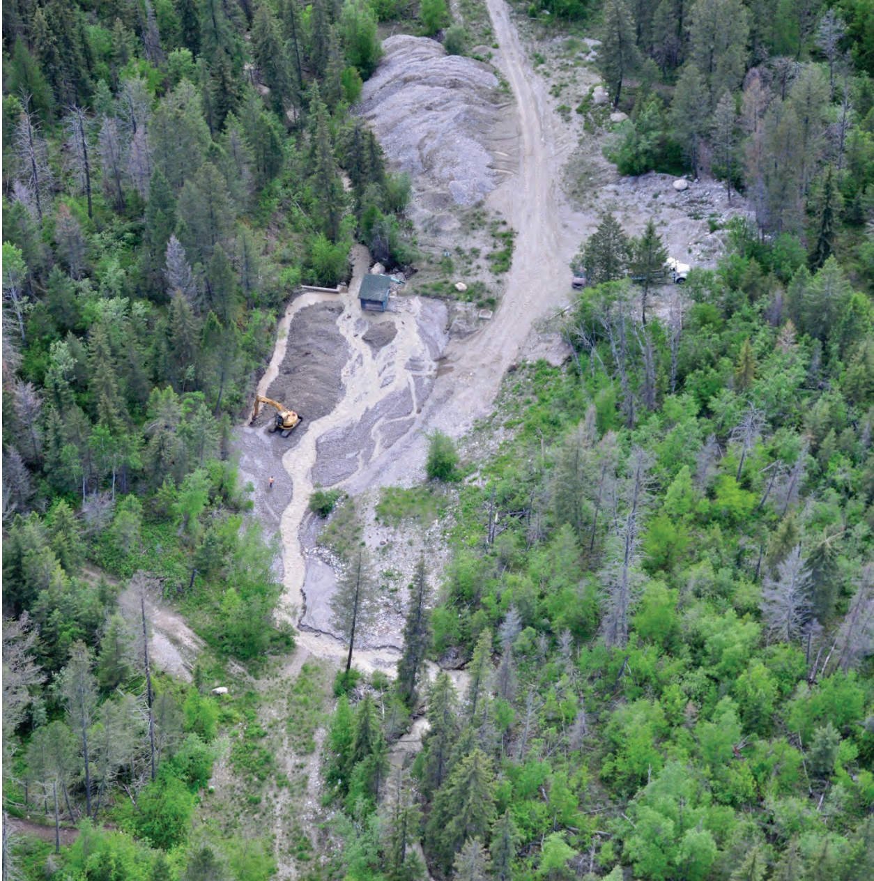
Photo 3.42 Sediment deposited in dam on Cold Spring Creek.
