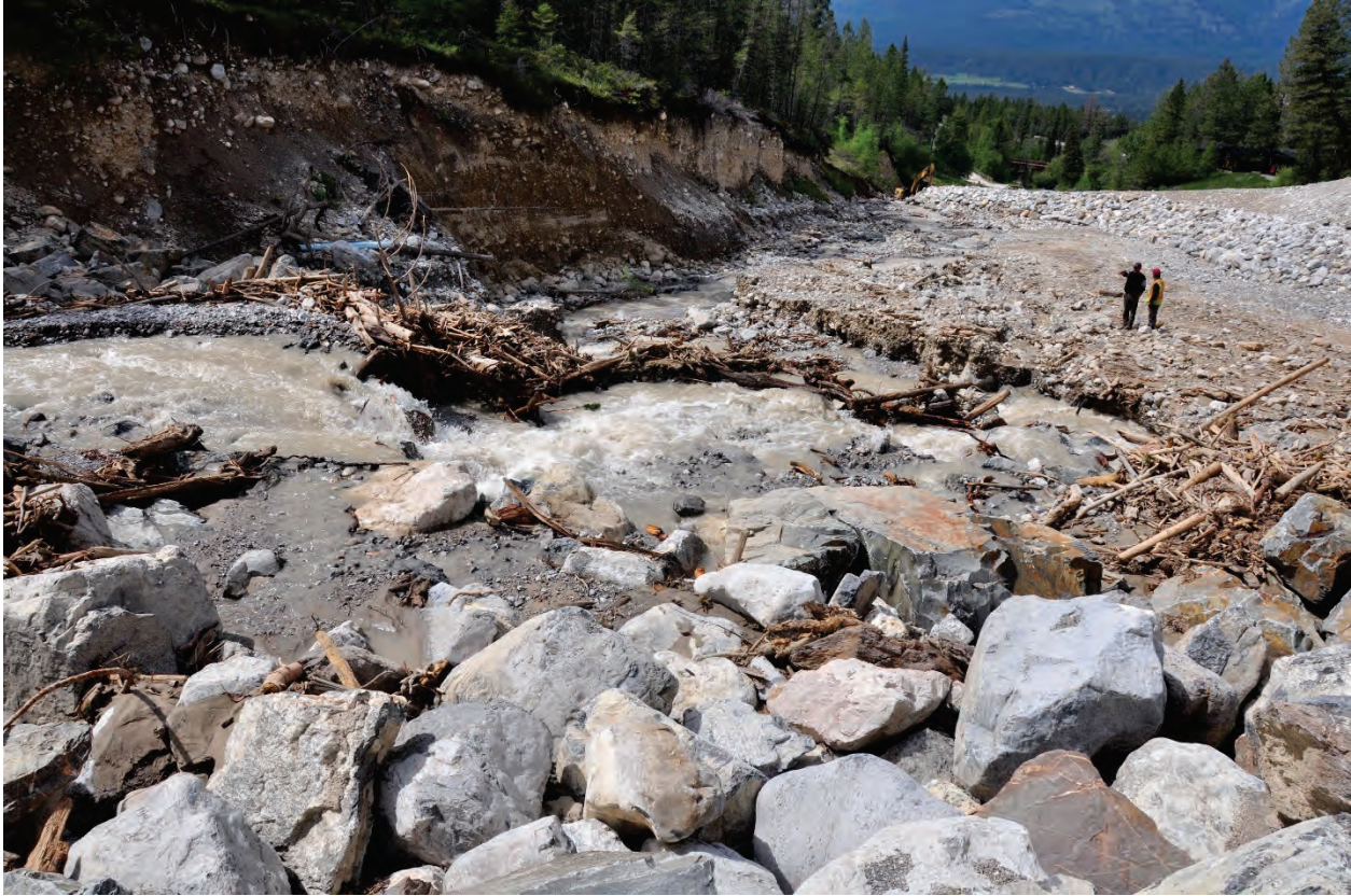
Photo 3.21 Sediment and debris that has passed overtop of weir # 3 is illustrated in foreground while scoured bed downstream of weir # 3 is also visible.
