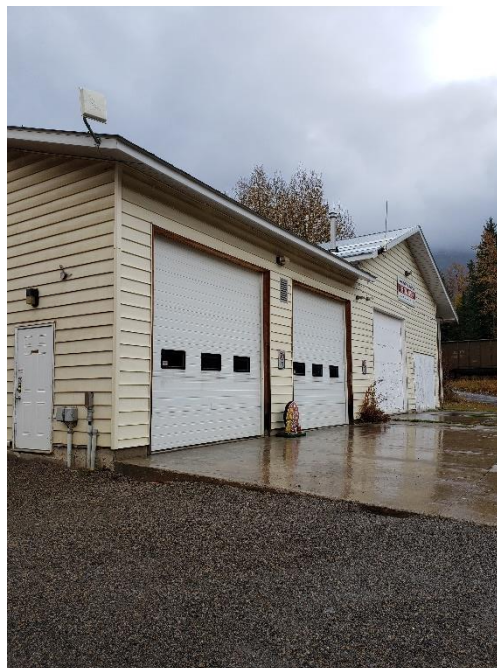
Figure 2: The current Hosmer Fire Station has a busy rail line along the rear property line and abuts known high-risk flood and inundation zones.
