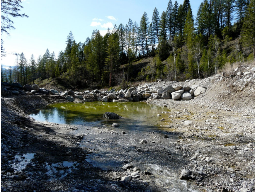
Photo 5: Debris Trap 2 View from Upper Section & US Slope of Weir
