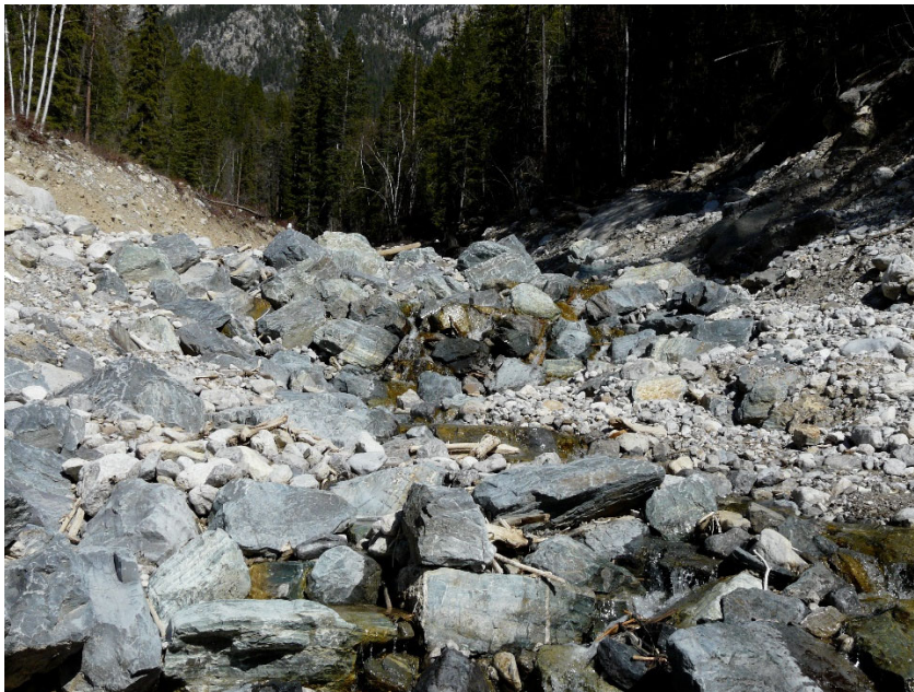
Photo 3: Debris Trap 1, Downstream Slope Looking Upstream
