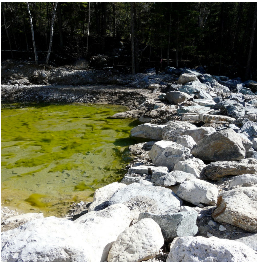
Photo 6: Debris Trap 2 US Slope of Weir
