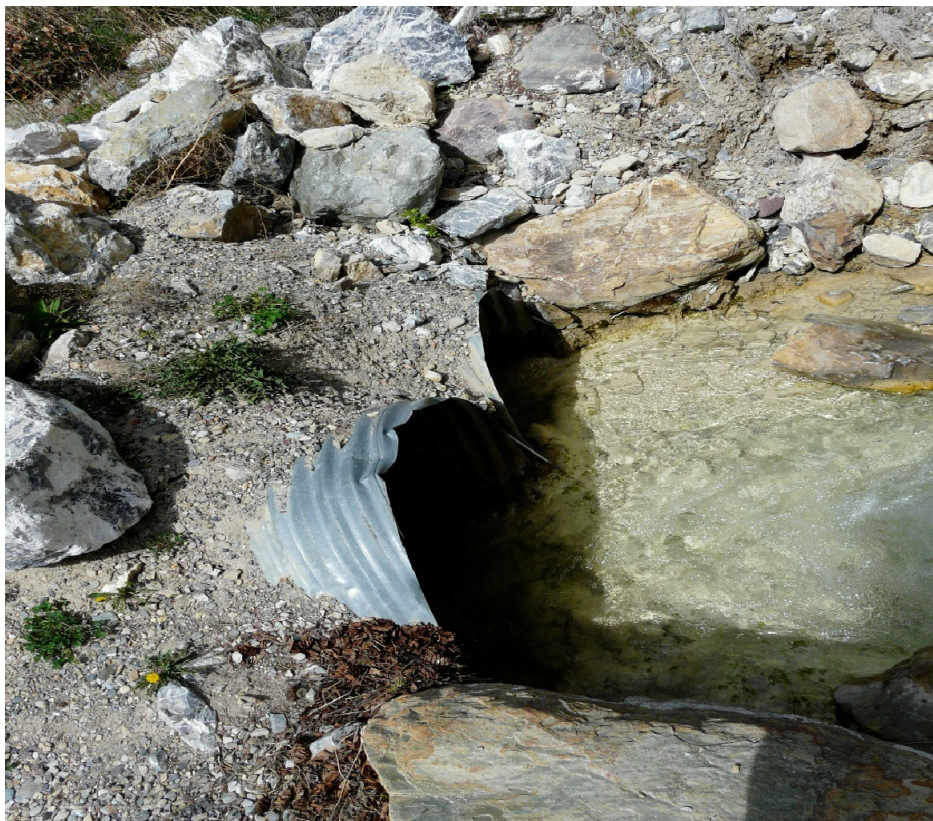
Photo 18: MoTI Culvert Infilling
