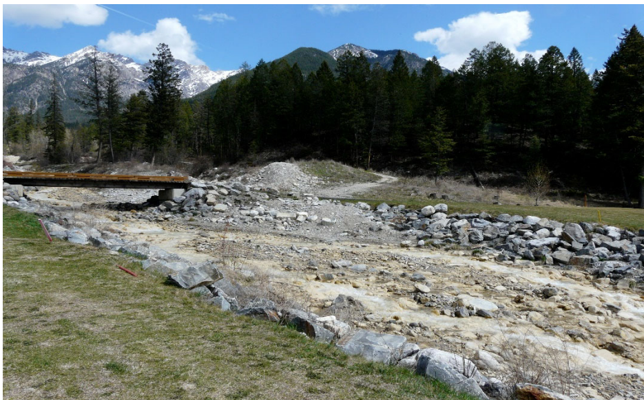
Photo 13: Left Bank Exposed Area Below Hole 16 Bridge. Possible equipment entry point
