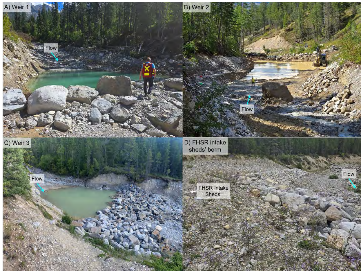
Figure 1-4 Photos of the weirs and berm taken during BGC's August 2024 field visit. The photo of the berm shows the general condition and structure of the berm but does not show the entire extent.
