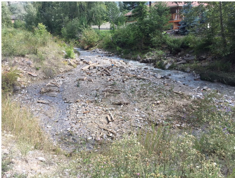
Photo 12: Small debris trap has some woody debris and minor debris flood deposition.
