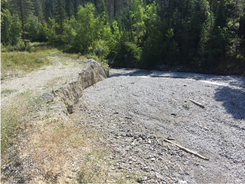
Photo 5: Cold Spring Creek Dam reservoir on August 21, 2019.
