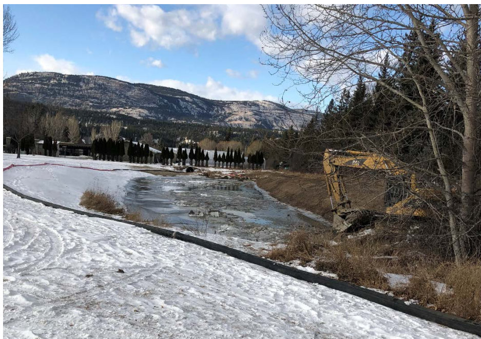
Photo 14: Cold Spring Creek lower debris trap. Photo taken December 19, 2019.
