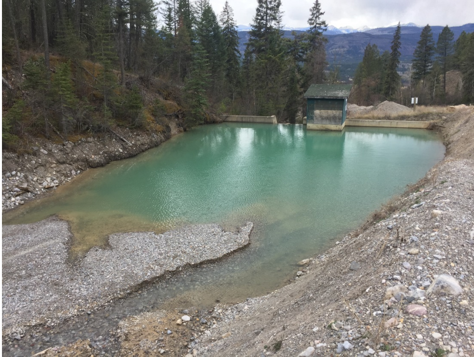
Photo 1: Cold Spring Creek Dam Reservoir, May 1, 2019.
