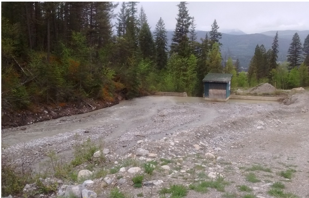
Photo 6: The Cold Spring Creek Reservoir was completely filled in by debris. Photo taken May 12, 2017.
