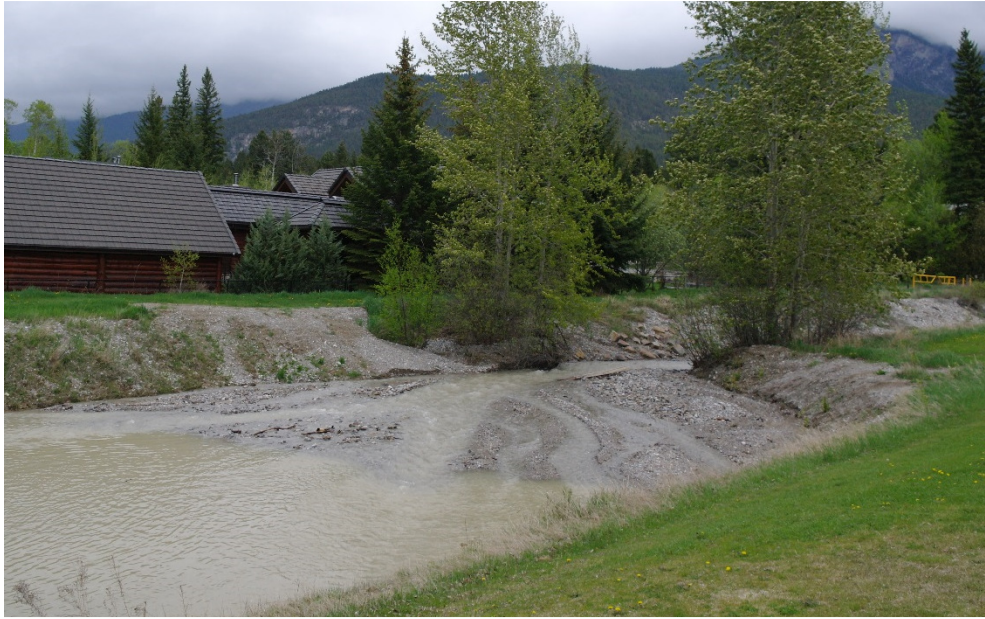
Photo 5: Material deposited at the entrance to the lower debris trap. Photo taken May 12, 2017.
