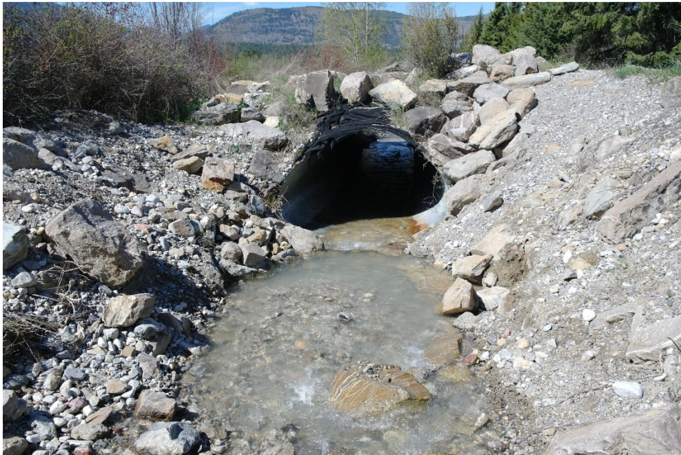
Photo 1: Inlet of the culvert above the debris pond, May 4, 2017.
