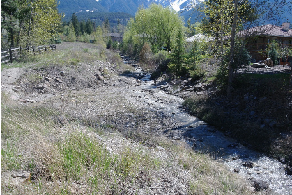
Photo 4: The mid-channel debris trap, May 4, 2017.
