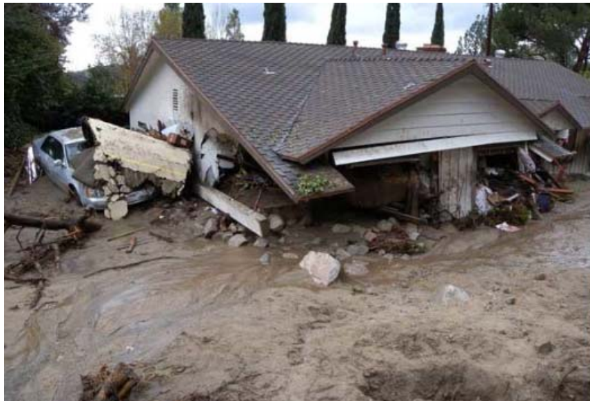
Figure E-1-1. Home damaged by debris flow at Montecito, California in January of 2018. Photo by USGS (public domain), https://www.usgs.gov/media/images/1s-post-fire-debris-flow . This type of destruction is entirely possible and even likely at Cold Spring Creek in the future.
