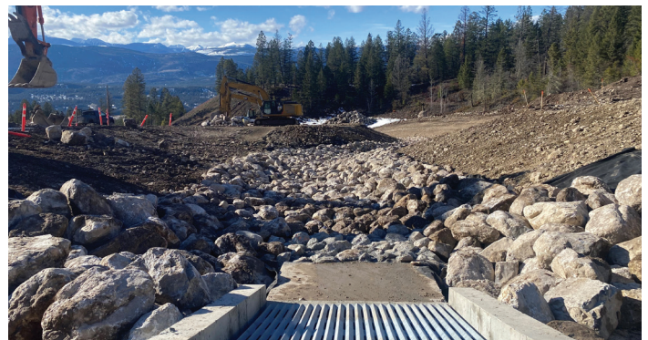
Photo: The new weir
