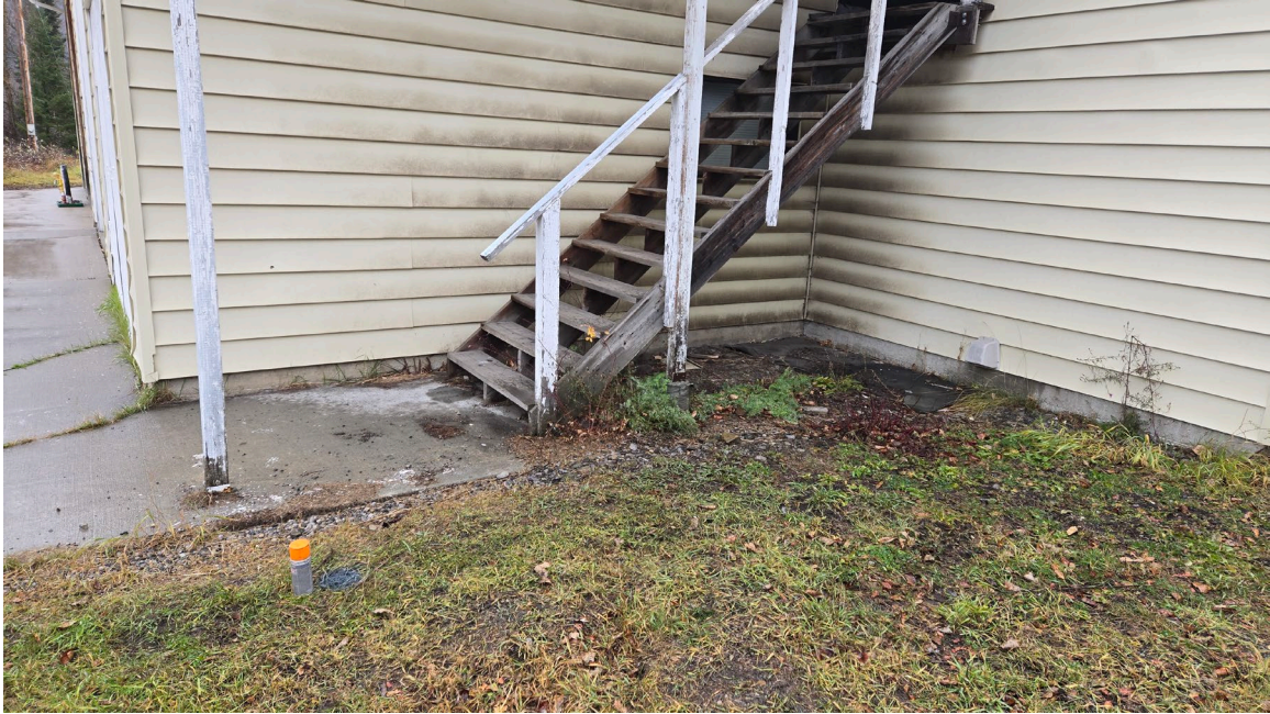
The end of the lateral is just to the right of the orange lid on the paint can.
