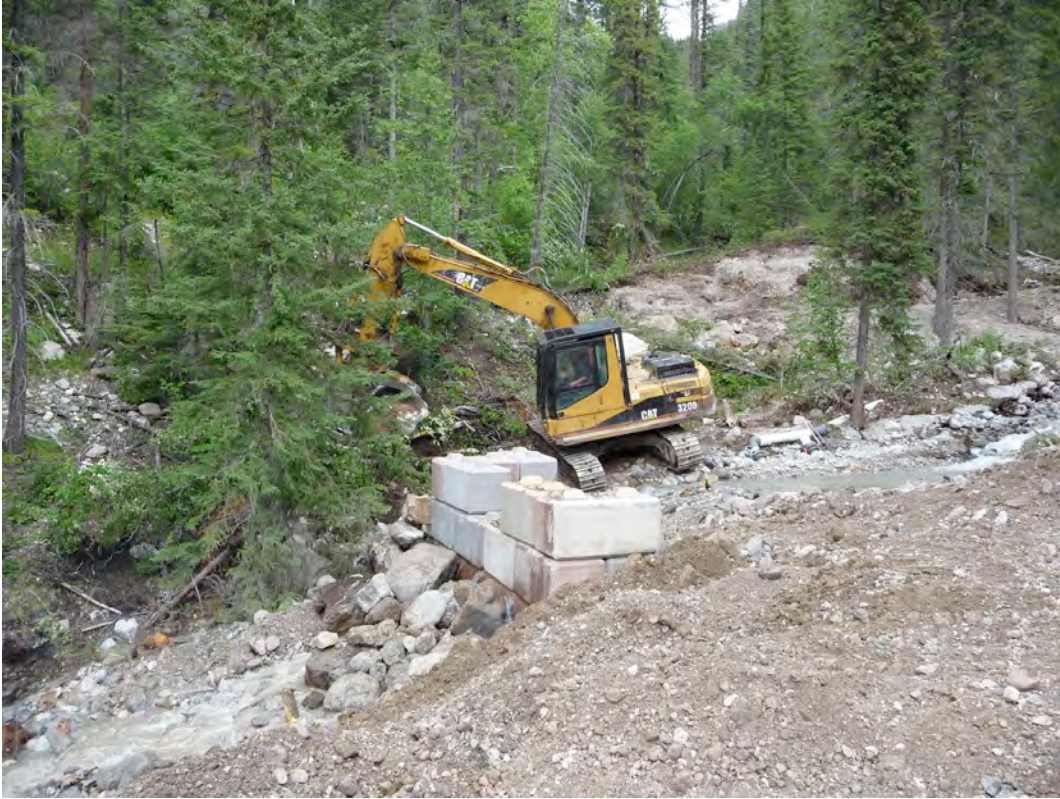
Photo 3: Reconstruction of water intake on Cold Spring Creek after 2011 event (exact date of photo unknown) (photo from RDEK)
