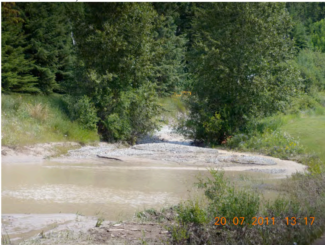
Photo 2: Sediment infilling of lower debris trap on Cold Spring Creek after flood event in 2011 (photo from RDEK)
