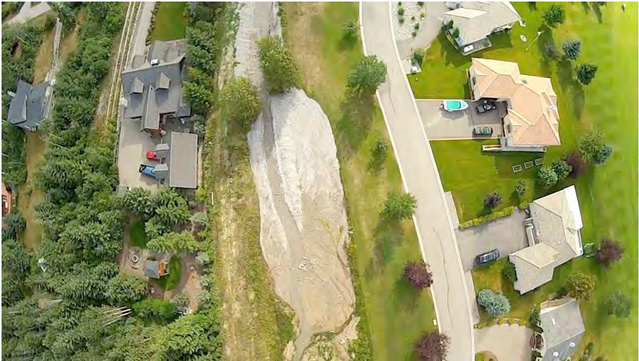
July 2013 Lower Reach of Cold Spring Creek showing partially infilled sediment basin
