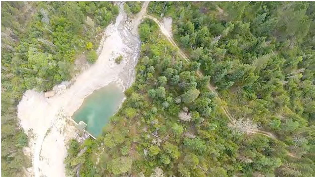
July 2013 Cold Spring Creek Dam
