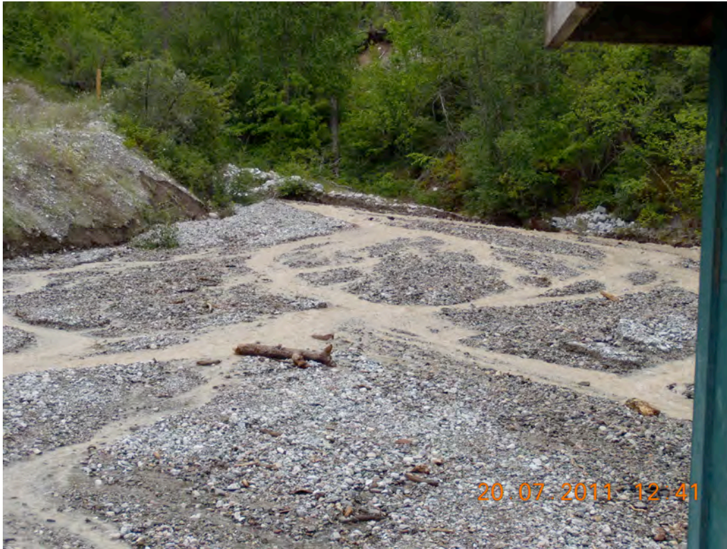
Photo 1: Sediment infilling of Cold Spring Dam reservoir after flood event in 2011 (photo from RDEK)
